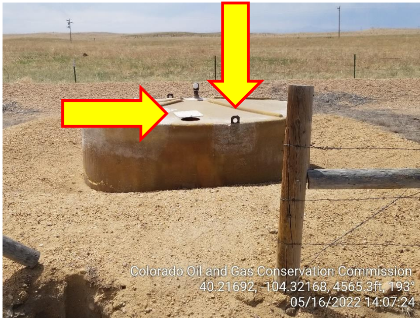
Photo 5 – Lid Open and Labels faded
