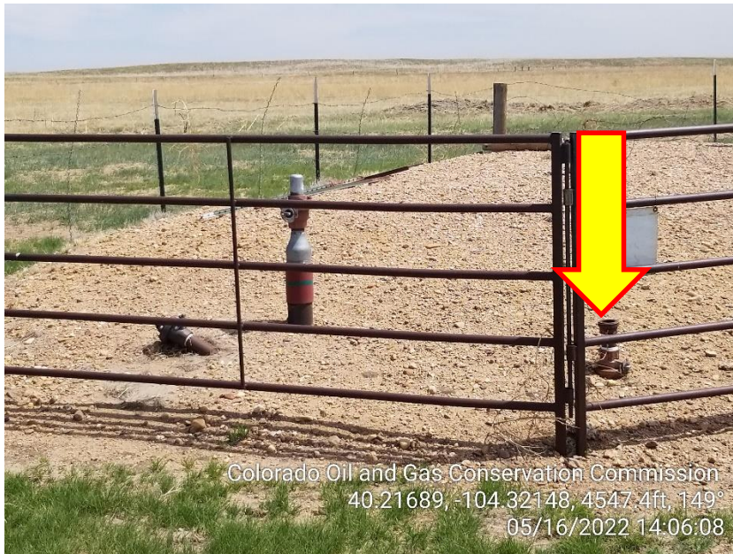
Photo 3 – Unmarked Riser at Wellhead
