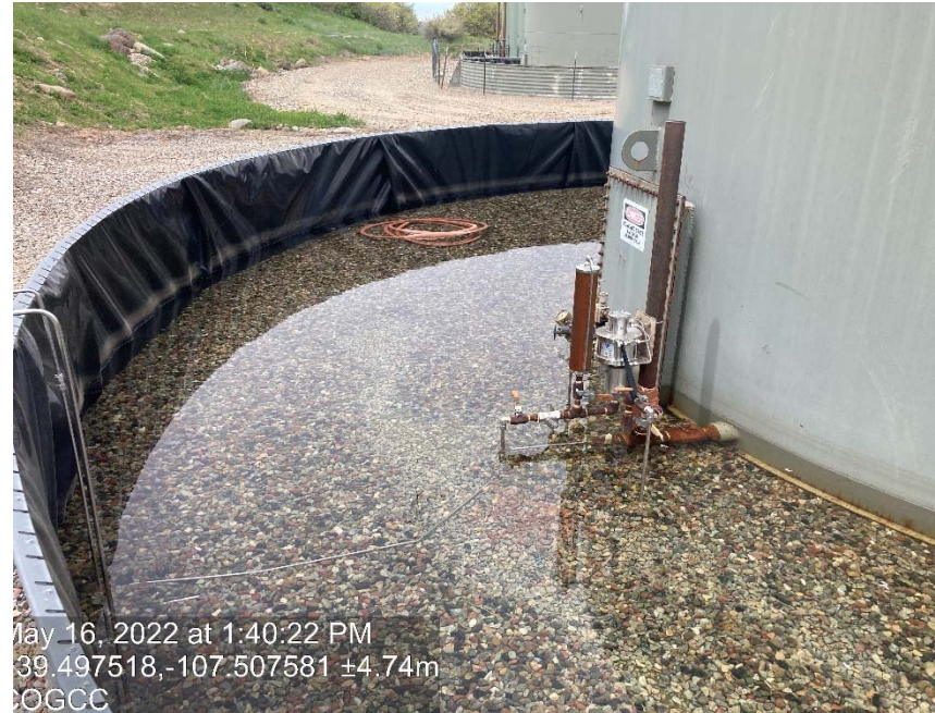
Tank containment with fluid
