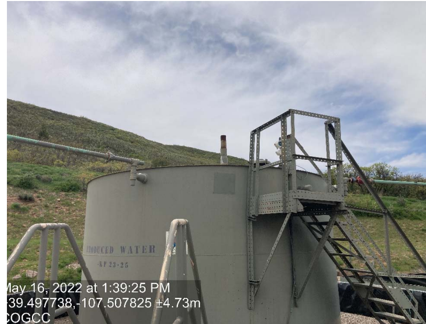
Production tank is open to atmosphere (venting)
