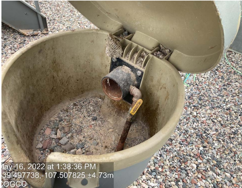
Valves on tanks missing caps/plugs
