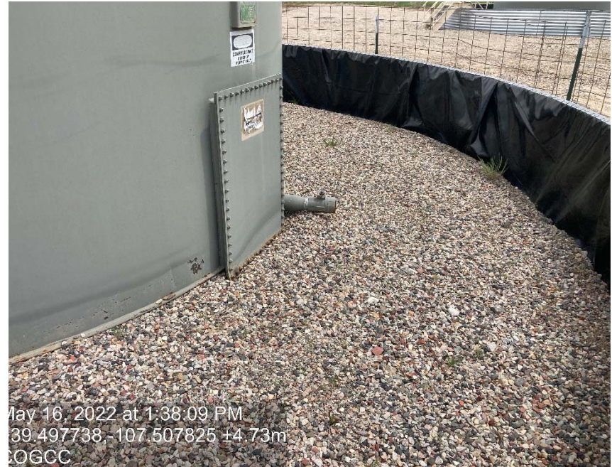
Valves on tanks missing caps/plugs
