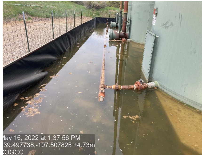
Tank containment with fluid
