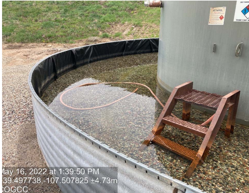
Tank containment with fluid
