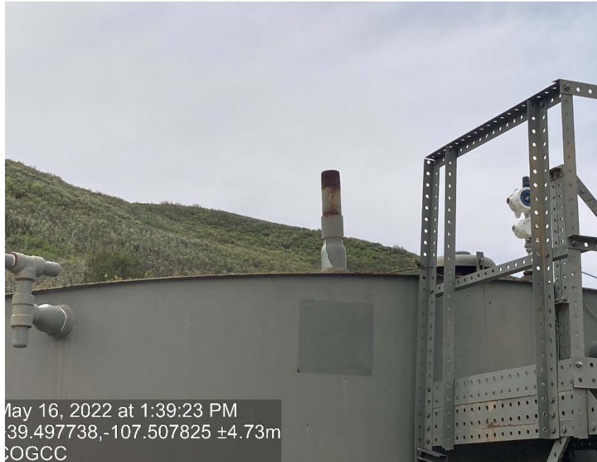
Production tank is open to atmosphere (venting)
