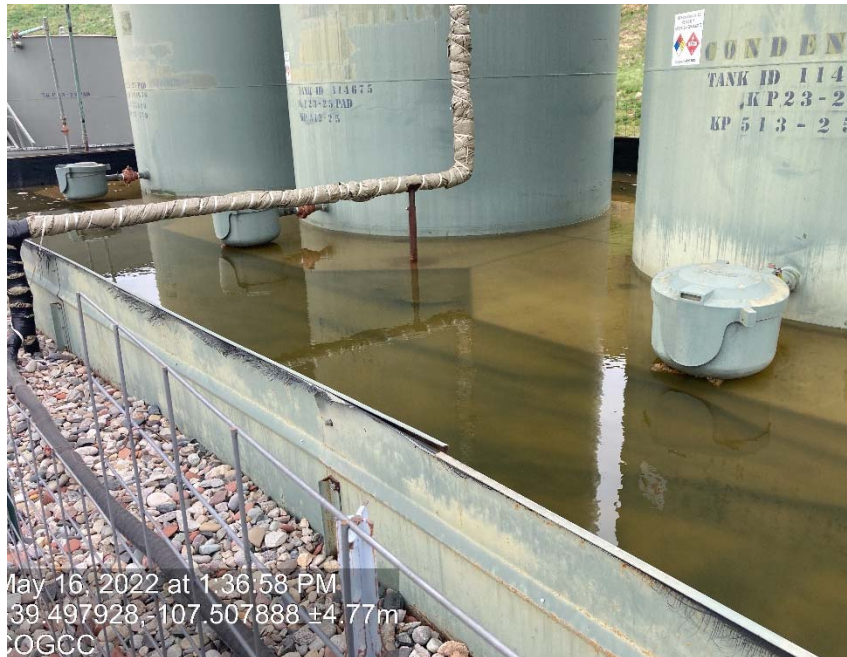
Tank containment with fluid
