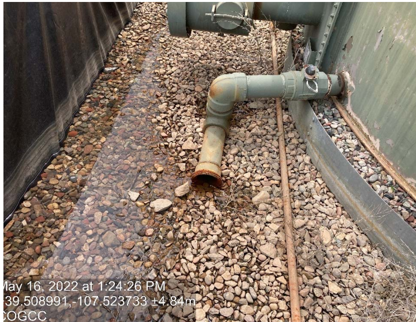
Valves on tanks missing caps/plugs
