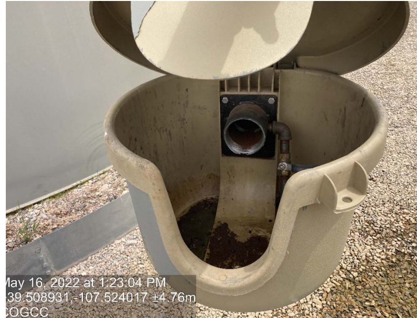
Valves on tanks missing caps/plugs
