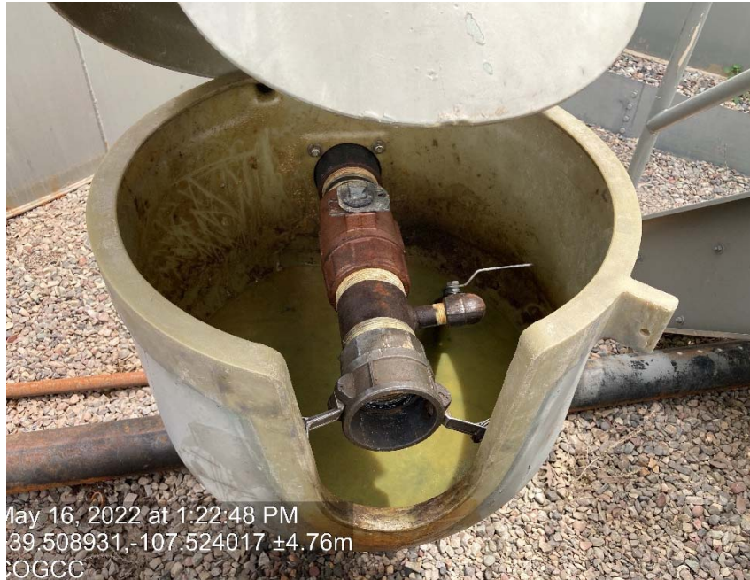
Valves on tanks missing caps/plugs
