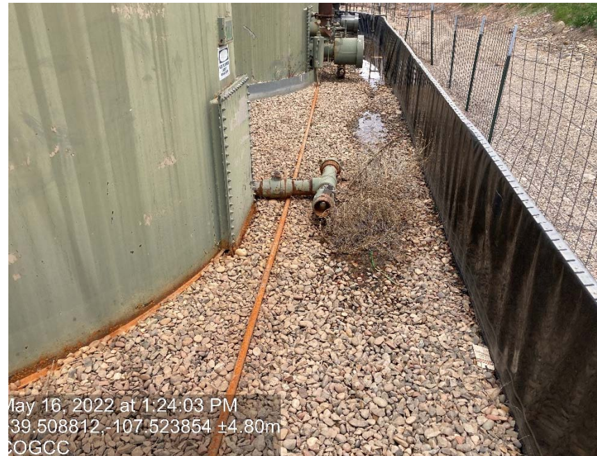
Valves on tanks missing caps/plugs and debris
