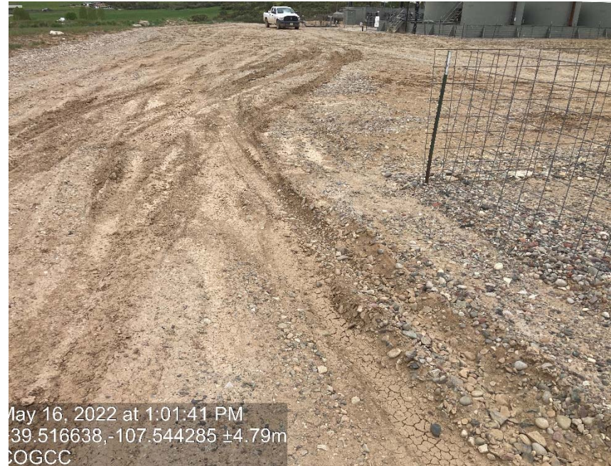
Lack of stabilization/compaction
