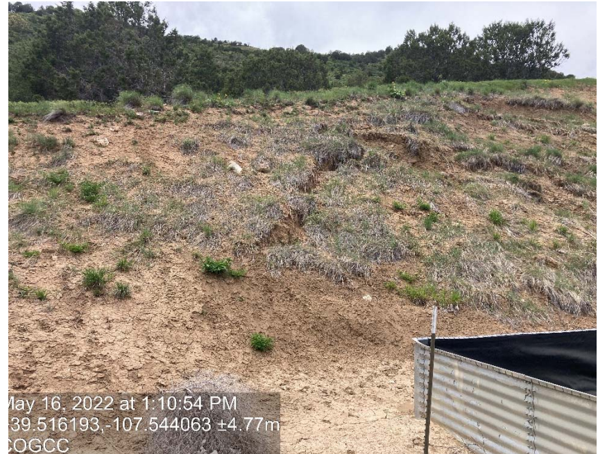
Cut slope erosion
