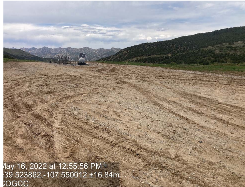
Lack of stabilization/compaction
