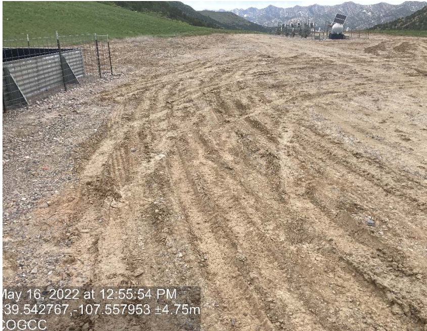
Lack of stabilization/compaction
