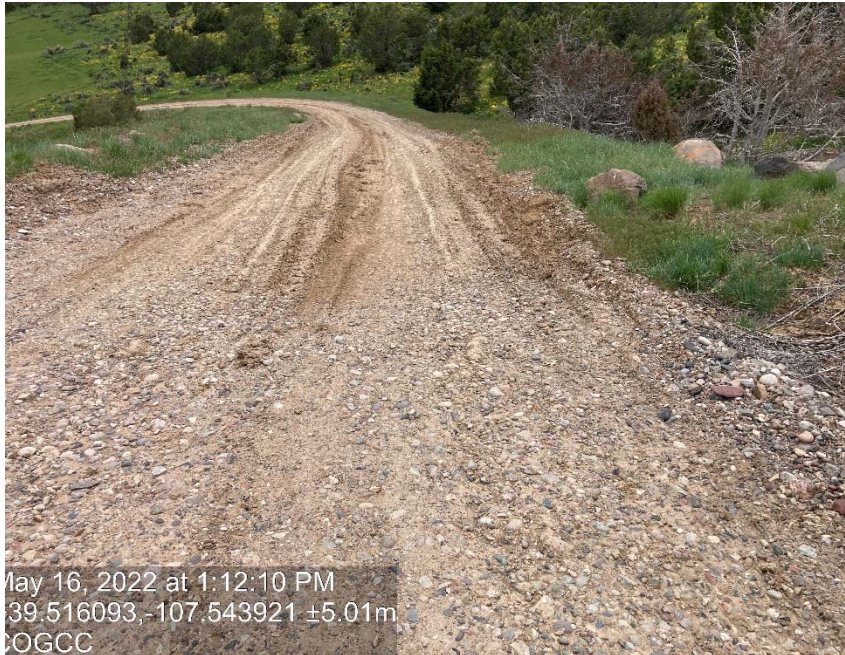
Lack of stabilization/compaction
