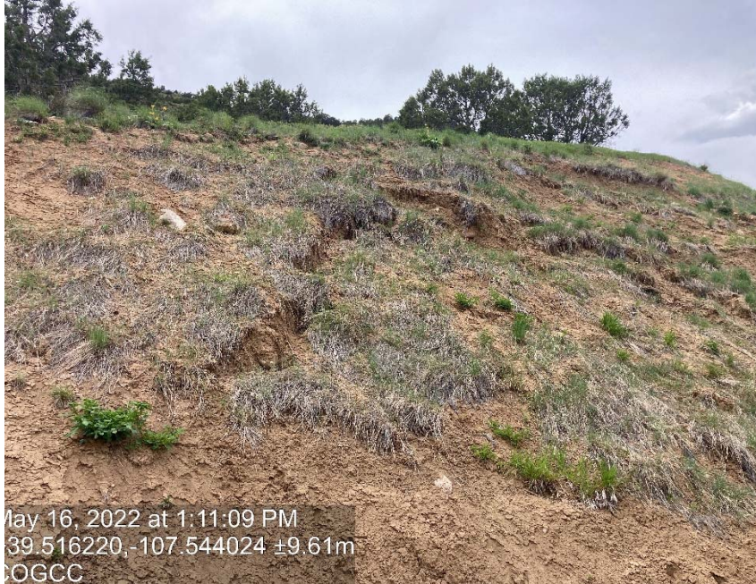
Cut slope erosion
