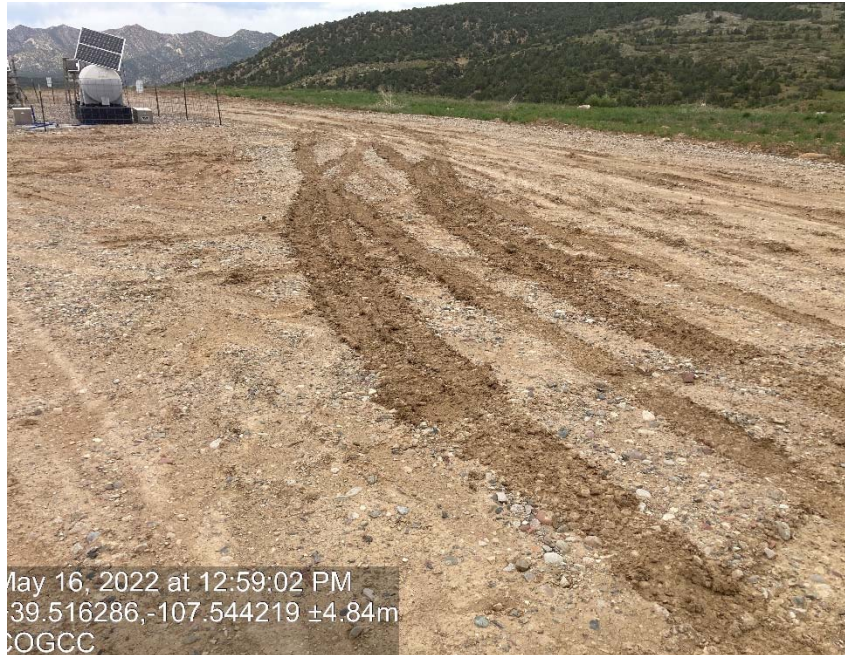
Lack of stabilization/compaction
