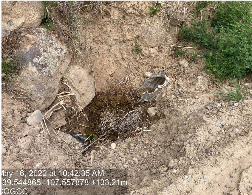
Access road inlet culvert is cleaned out from previous inspection
