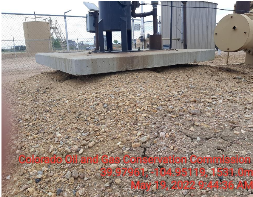
Photo 5 unsafe condition ECD cement base
