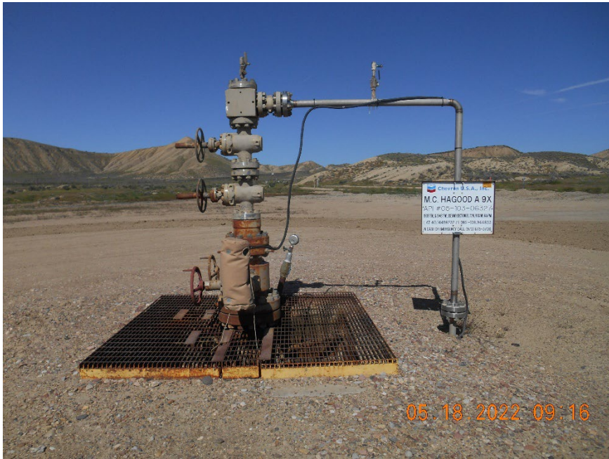
Injection wellhead
