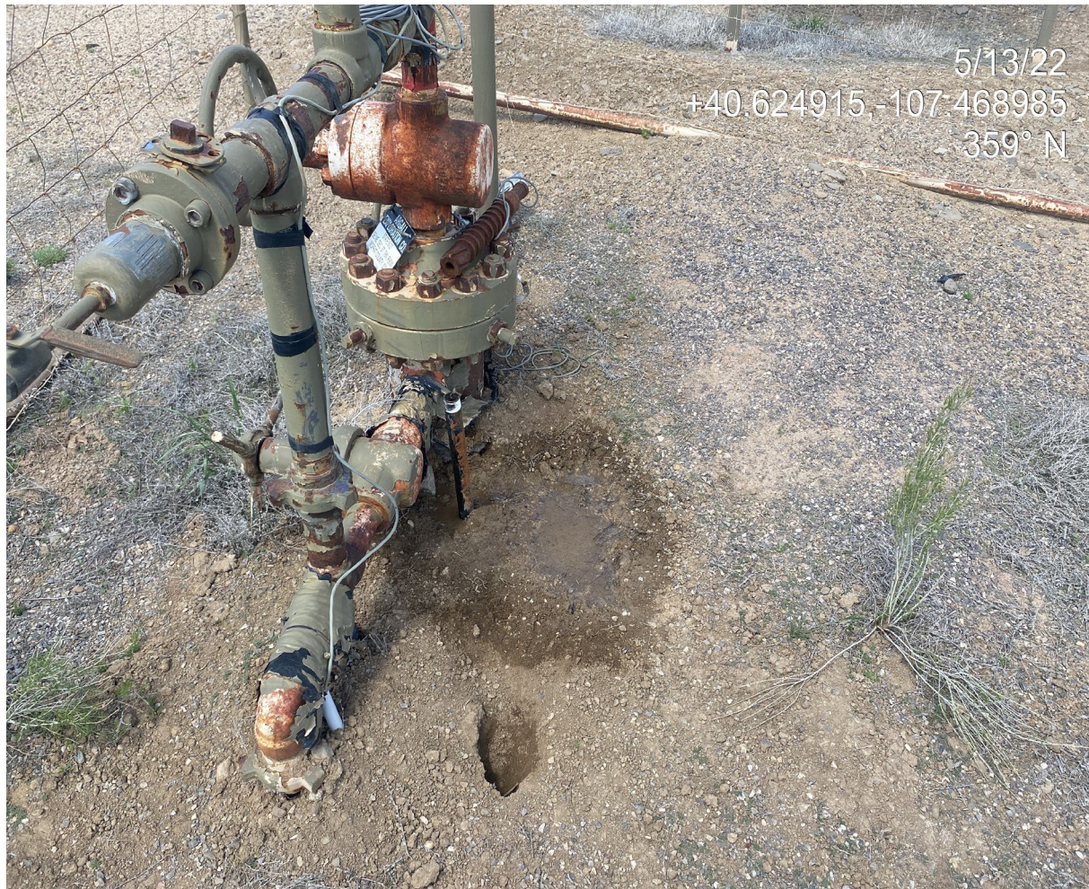
Photo 4. Photo taken from the wellhead shows water and gas bubbling up through a pipe.
