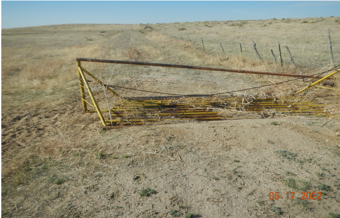
Photo 1. Facing south toward the access road. The cattleguard has not been removed and is filled in with sediment.
