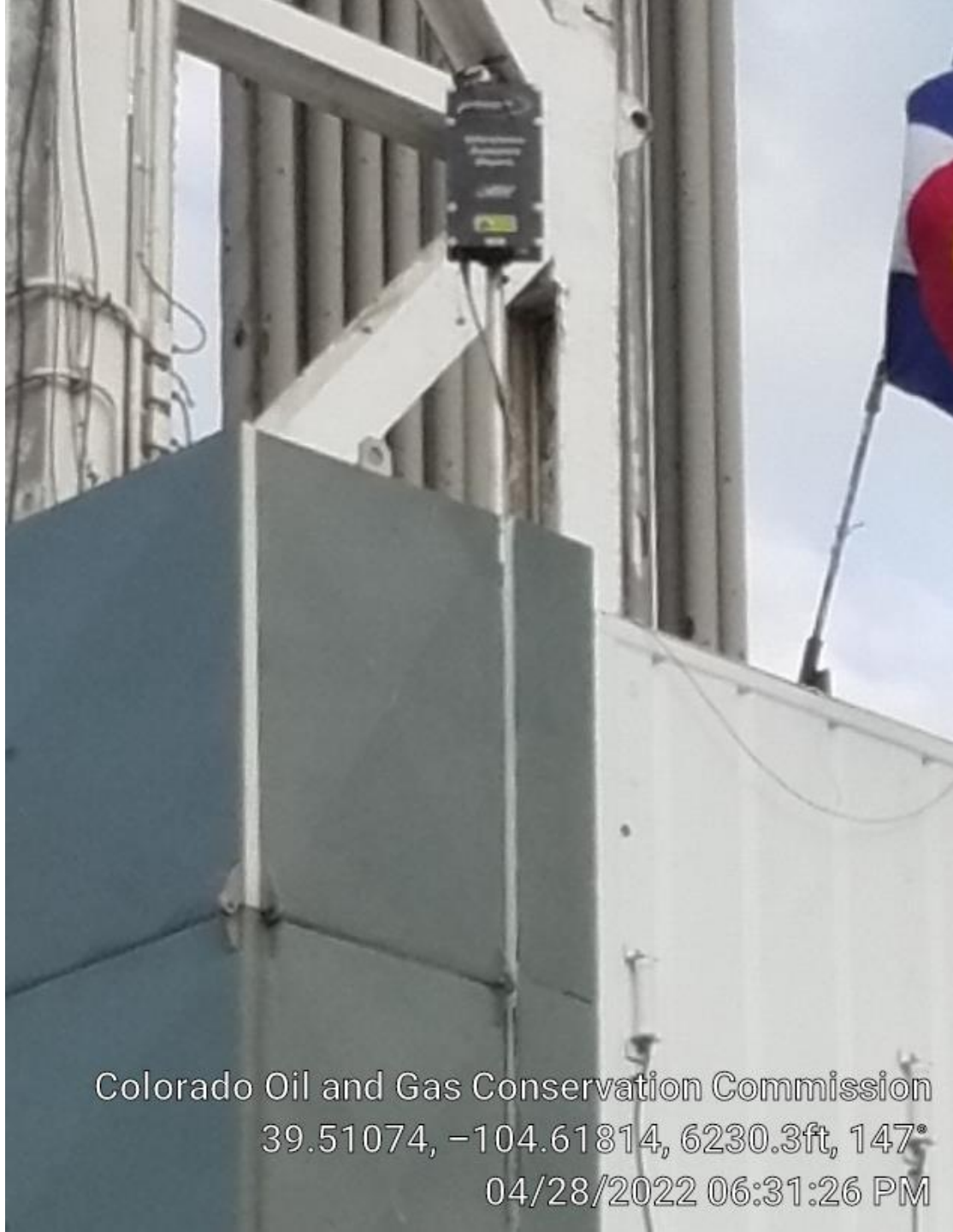
Monitoring equipment on rig
