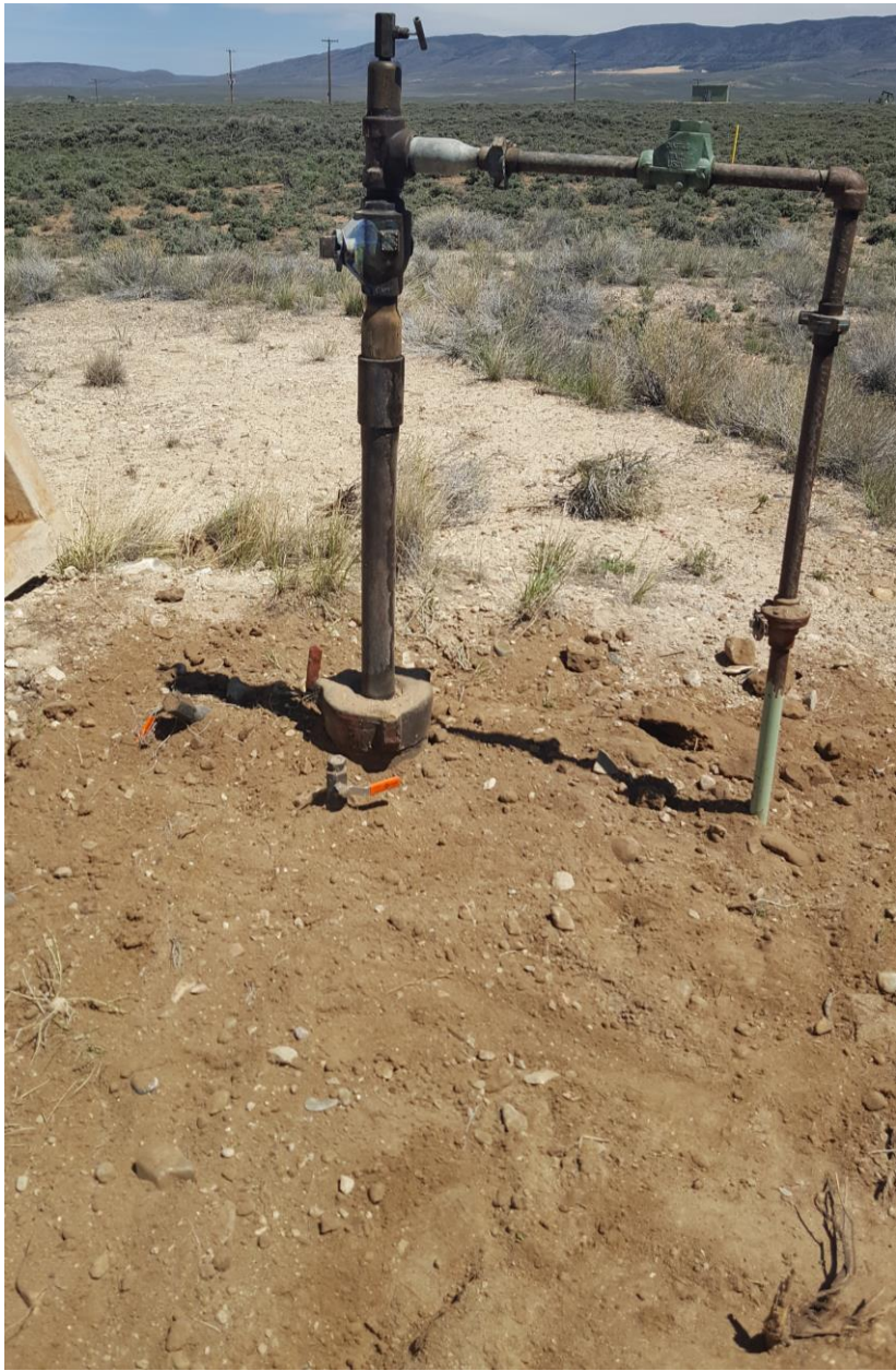
Figure #1 Bradenhead access has been installed.
