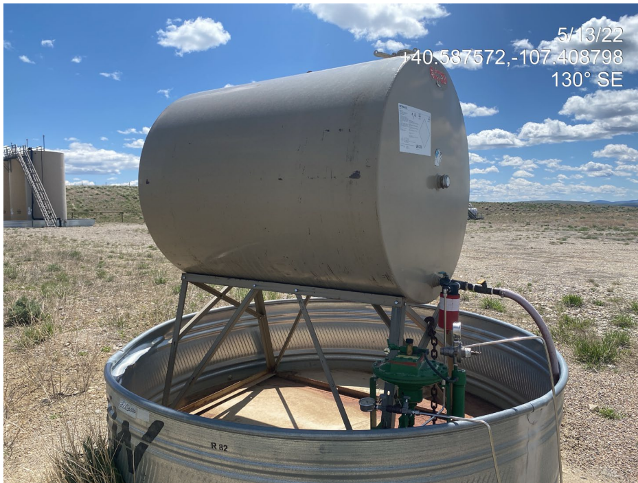
Photo 5. Photo taken from the north of the Location shows a methanol tank secondary containment stock tank lacking wildlife protection BMPs.
