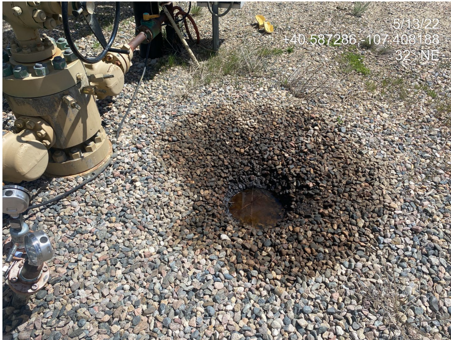
Photo 7. Photo taken from the wellhead shows an open casing.
