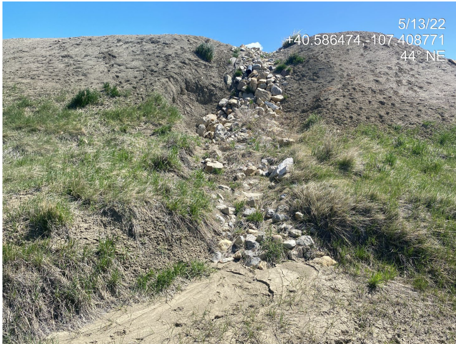
Photo 14. Photo taken from the southwest of the Location shows where a stormwater pipe is not properly designed or maintained in proper functioning condition. Stormwater has incised the berm around the pipe resulting in a large gully.
