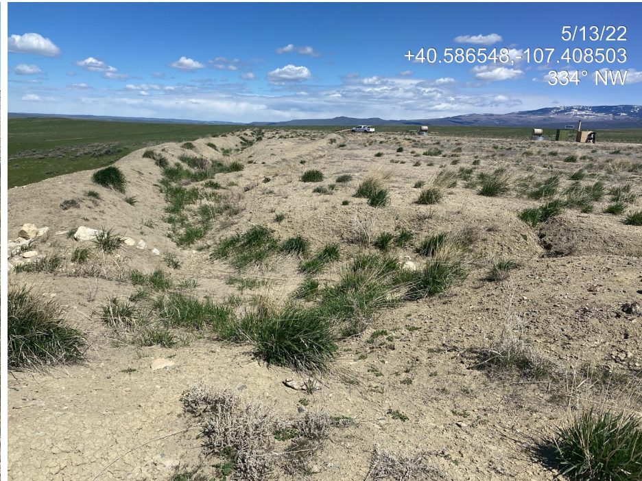
Photo 15. Photo taken from the southwest of the Location shows where perimeter ditches lead into a discharge pipe. Erosion of the pad in multiple directions leading into the ditch and pipe is evident.
