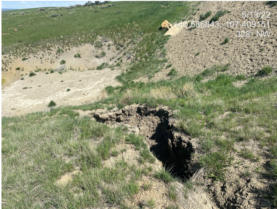
Photo 16. Photo taken adjacent from the west of the Location shows where a stormwater ditch is eroding and forming a gully.
