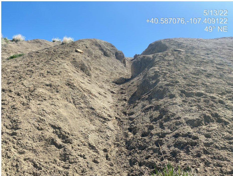
Photo 12. Photo taken from the west of the Location shows where a stormwater berm is not properly designed or maintained in proper functioning condition. Stormwater has incised the berm resulting in a large gully.
