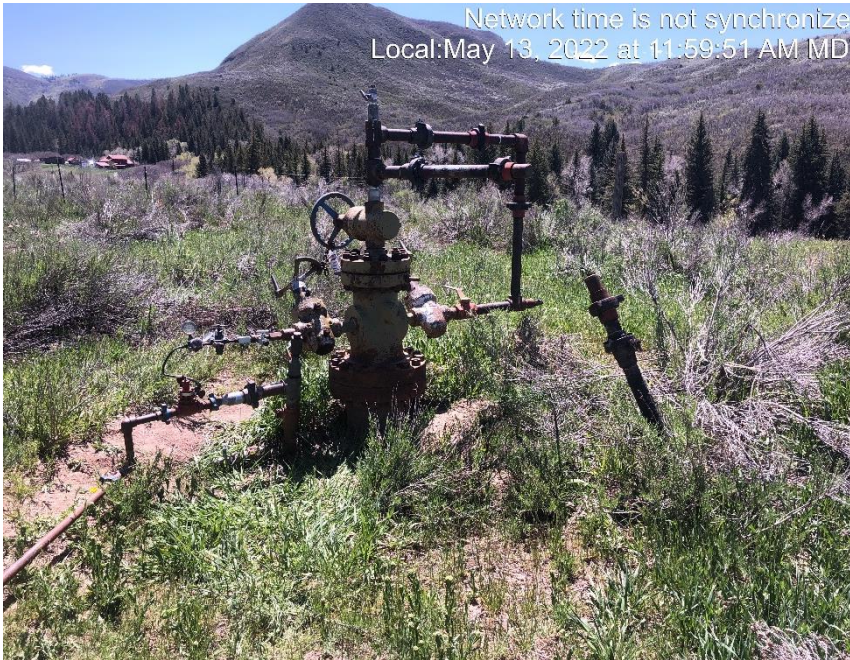
Photo #6705 No wellhead sign located at the well head.
