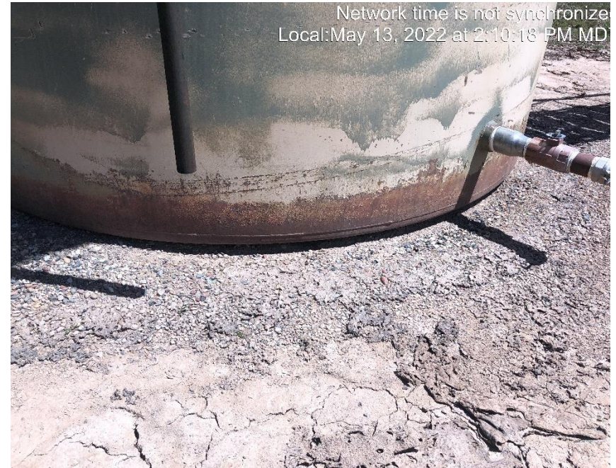
Photo #6720 Vent pipe on tank open.
