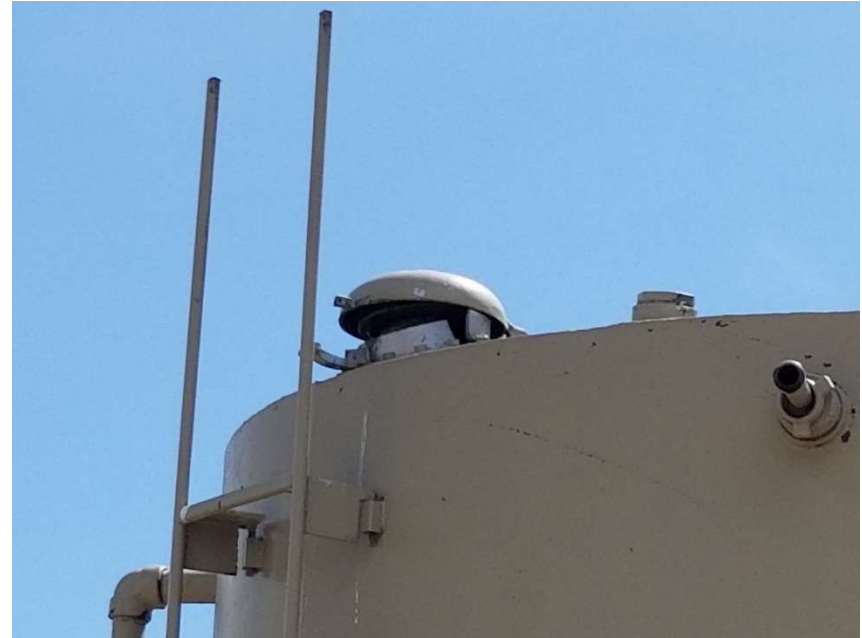
Photo 4. Close up of open gauge hatch.
