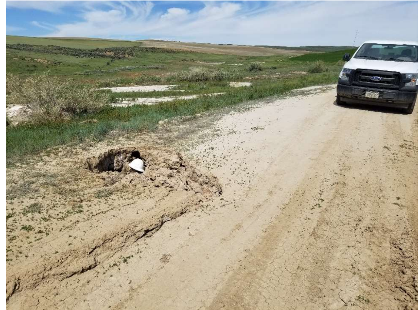
Photo 6. Collapse in access road. Hard hat for scale.
