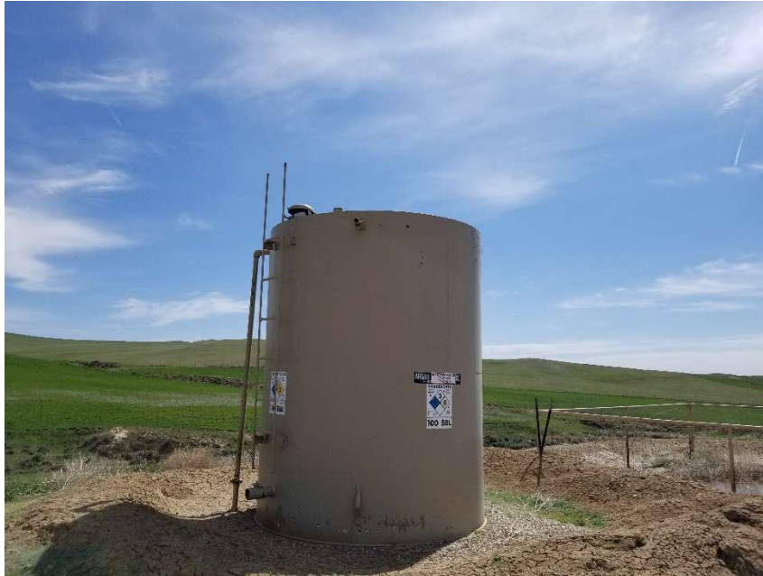
Photo 3. Gauge hatch open. Animal burrows in berm.
