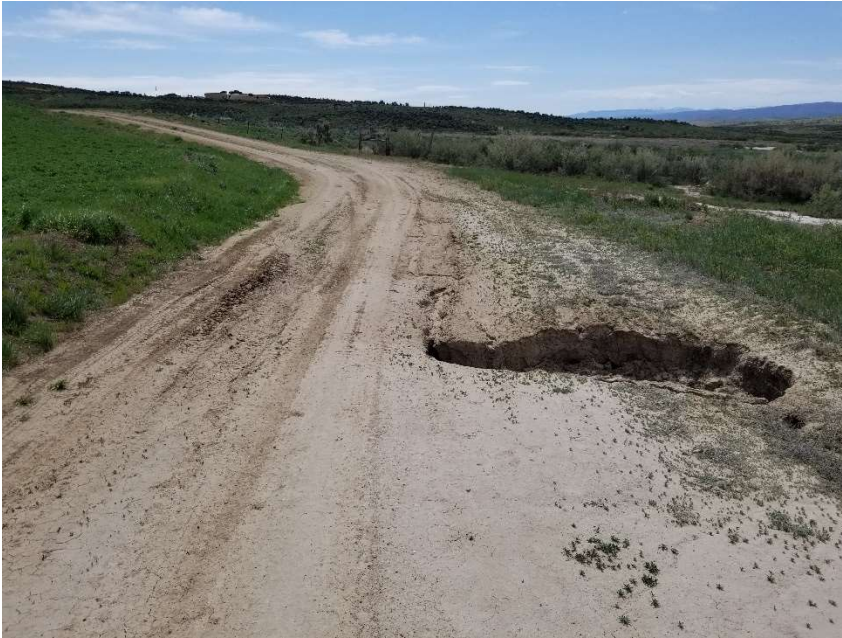
Photo 5. Collapse in access road.
