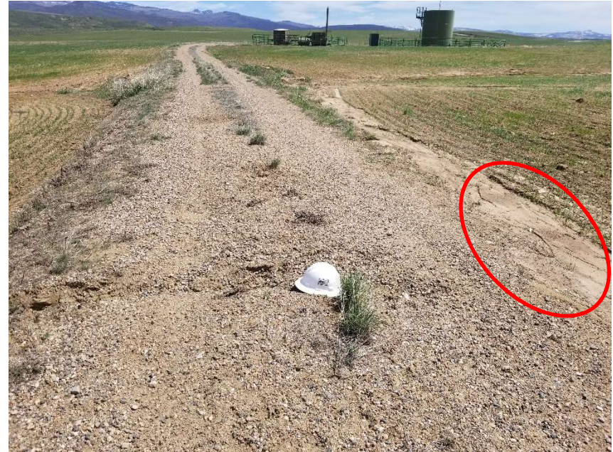
Photo 6. Sediment migration onto and across access road.
