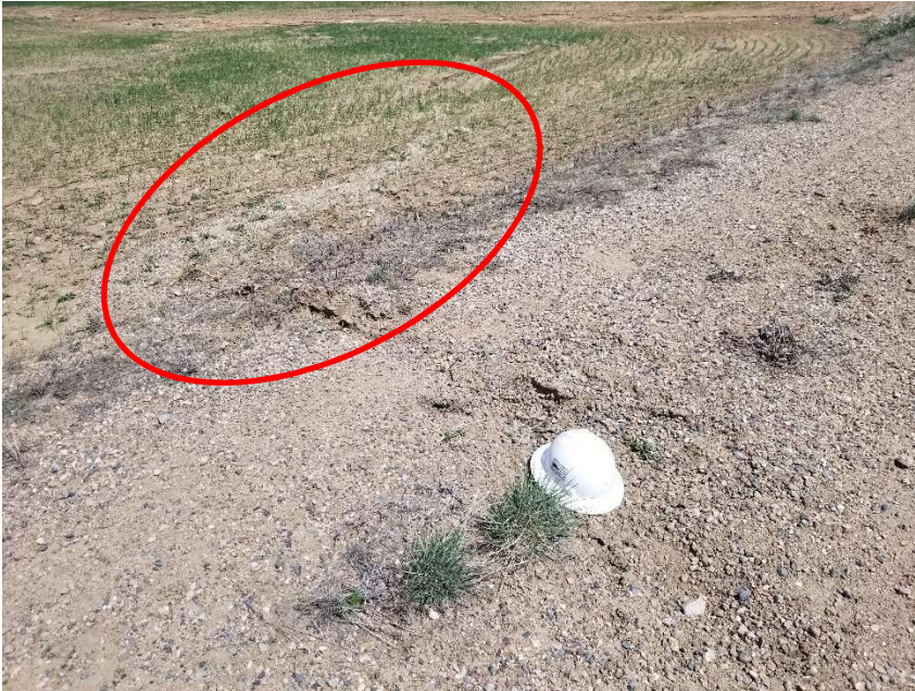
Photo 5. Sediment migration across and off access road. Hard hat for scale.
