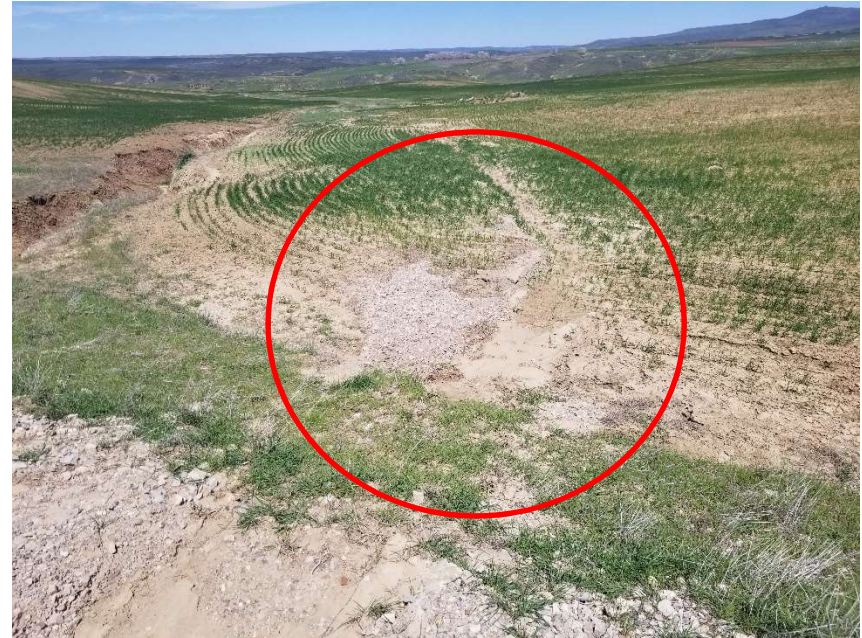
Photo 6. Close up of sediment transported off of access road.
