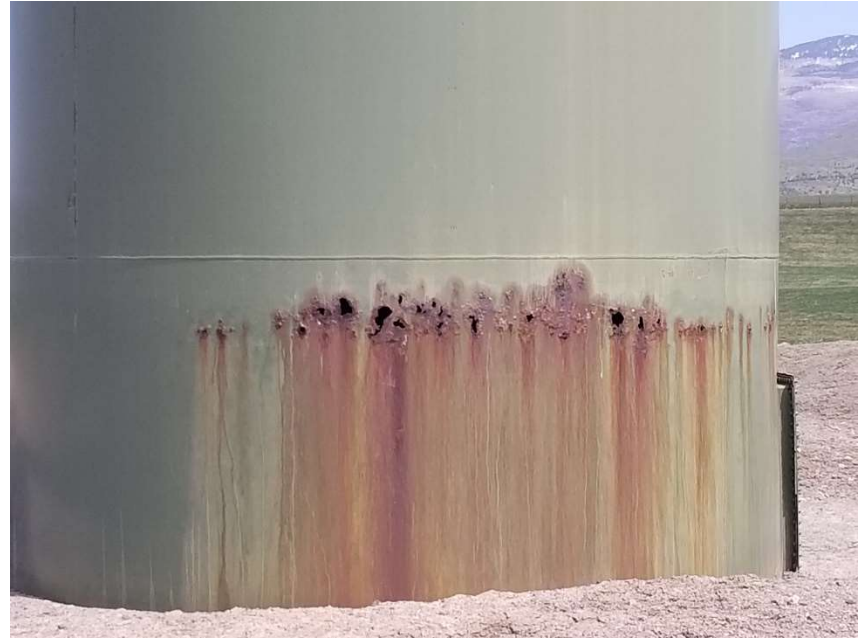
Photo 10. Close up of holes in produced water tank.
