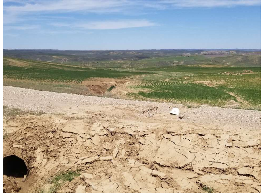
Photo 4. Culvert with road damage. Hard hat for scale.
