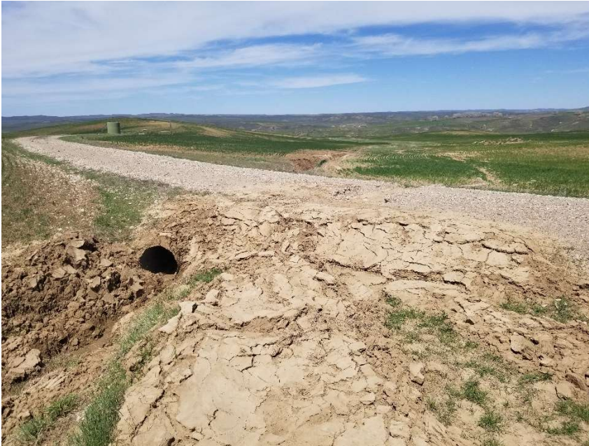
Photo 3. Culvert that appears damaged or overwhelmed.
