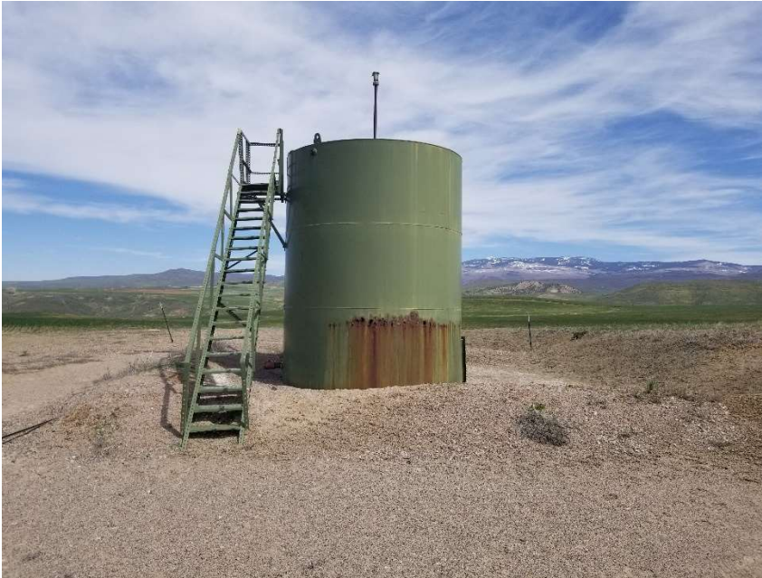
Photo 9. Holes in produced water tank.
