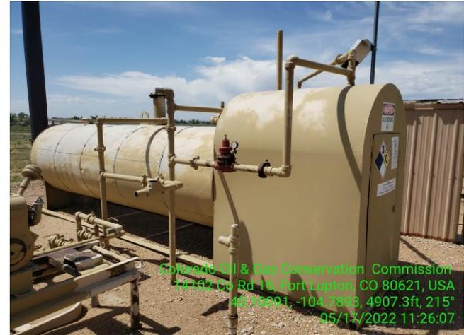
**Photo 7 Gas Meter Run, No card to indicate calibration status.**
