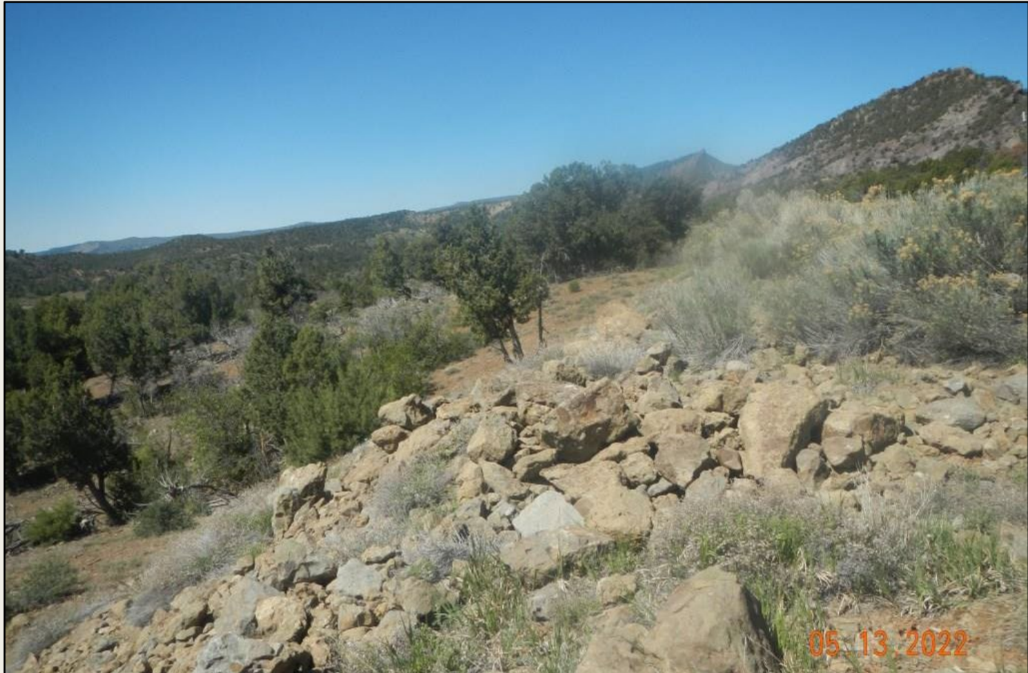
Photo 2. View of the southern fill slope from the southeastern corner facing westward. Slope is largely rock stabilized with western wheatgrass, rubber rabbitbrush, hairy goldenaster, and crested wheatgrass observed.
