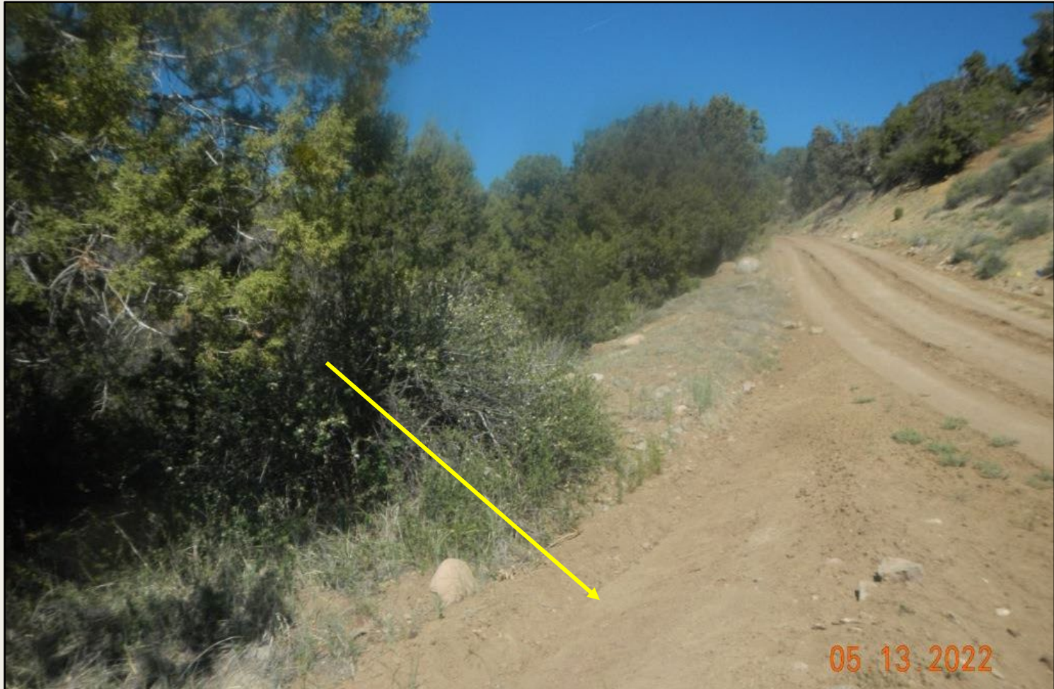
Photo 6. View of unstabilized turnout (yellow arrow) with loose soils and stormwater BMPs not present.
