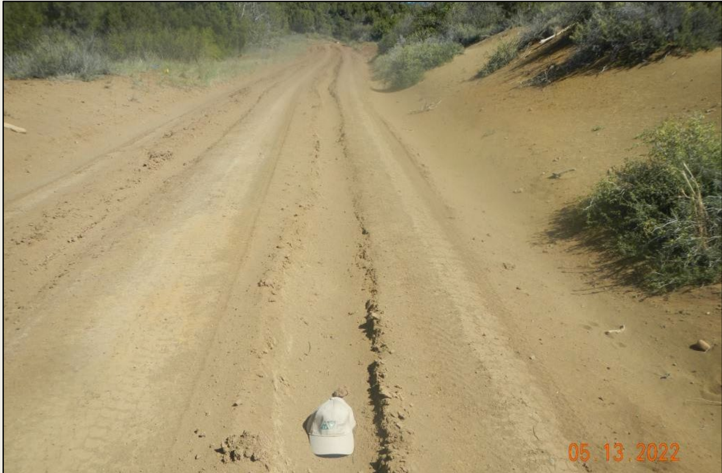
Photo 8. View of erosional channeling on access road surface, approx. 1-1.5ft wide and deep. Road surface is not stabilized.
