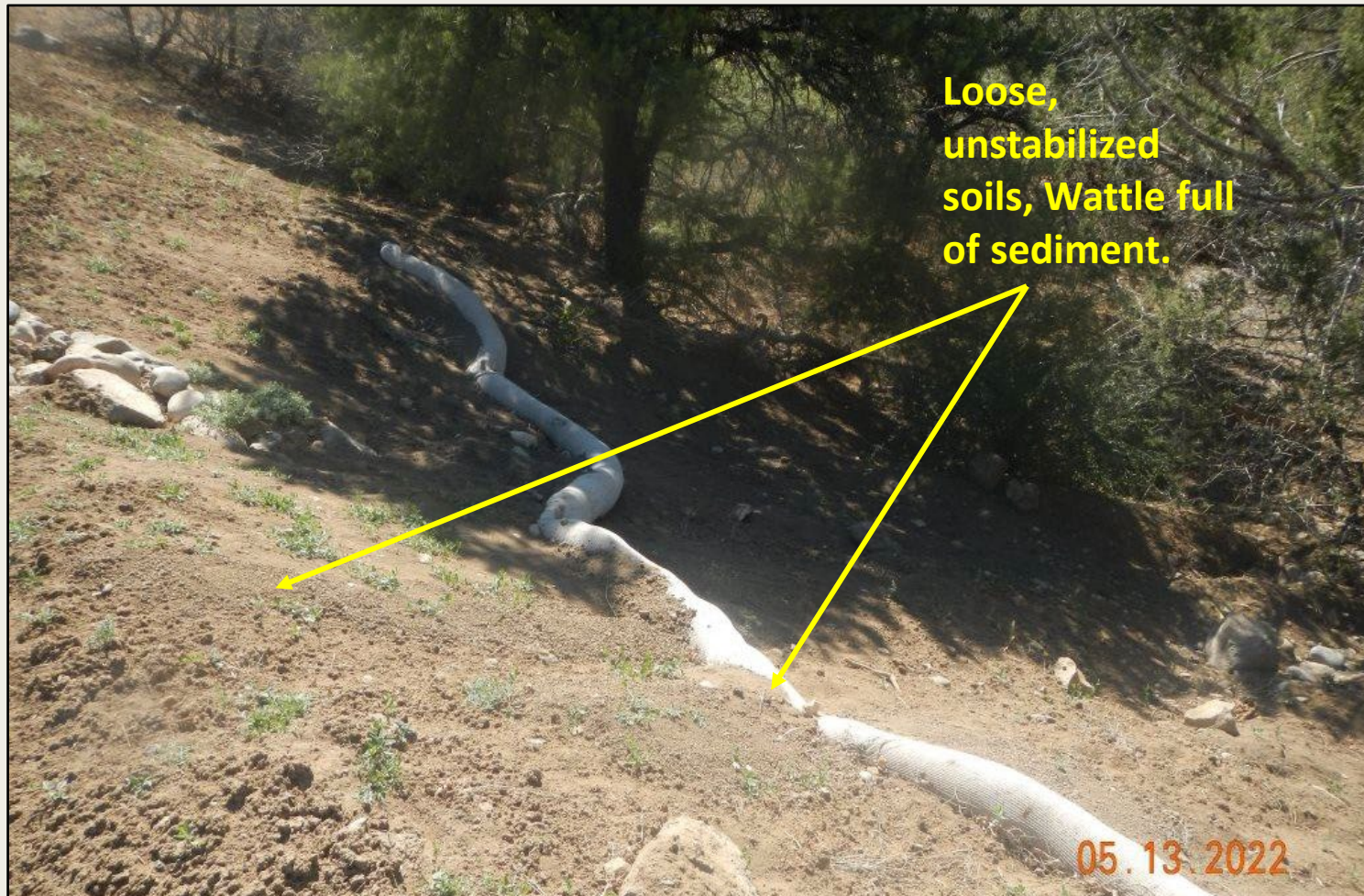
Photo 4. View of wattles down-slope from access road full of sediment and not functioning. Soils on slope are not stabilized.
