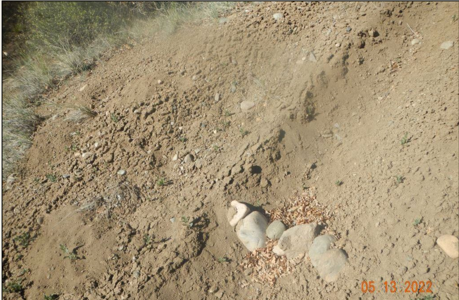
Photo 5. View of cobble installed along roadside surrounded by loose soils. This is not an appropriate nor adequate BMP to reduce stormwater erosion.
