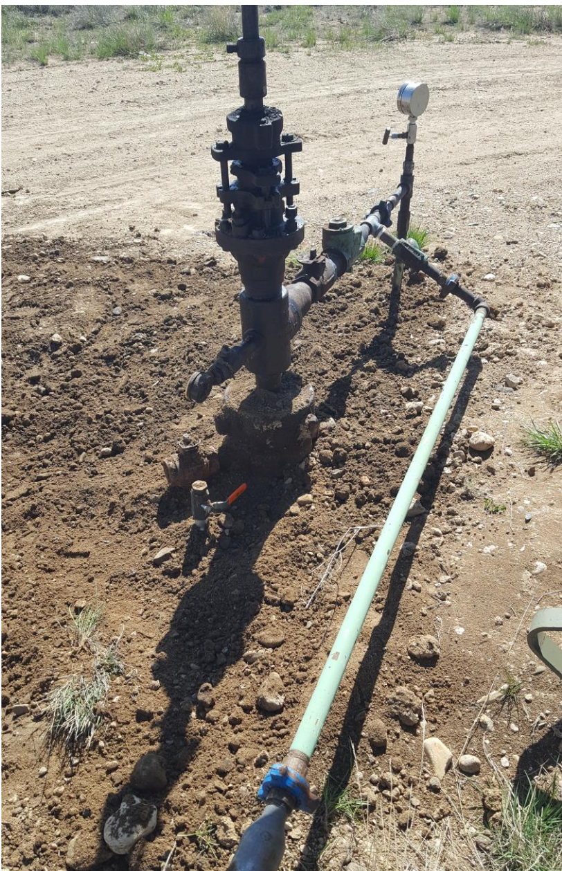
Figure #1 Bradenhead access has been installed.
