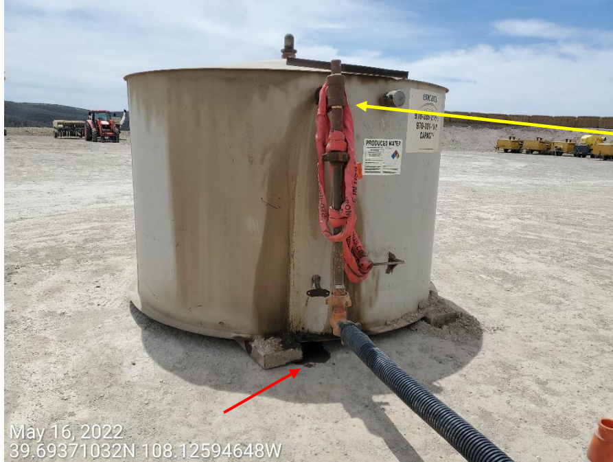
Photo 2: Fluids observed spilling from connection point of the line and tank (yellow arrow) onto the working pad surface. Stained soils also evident beneath the tank. (red arrow).
