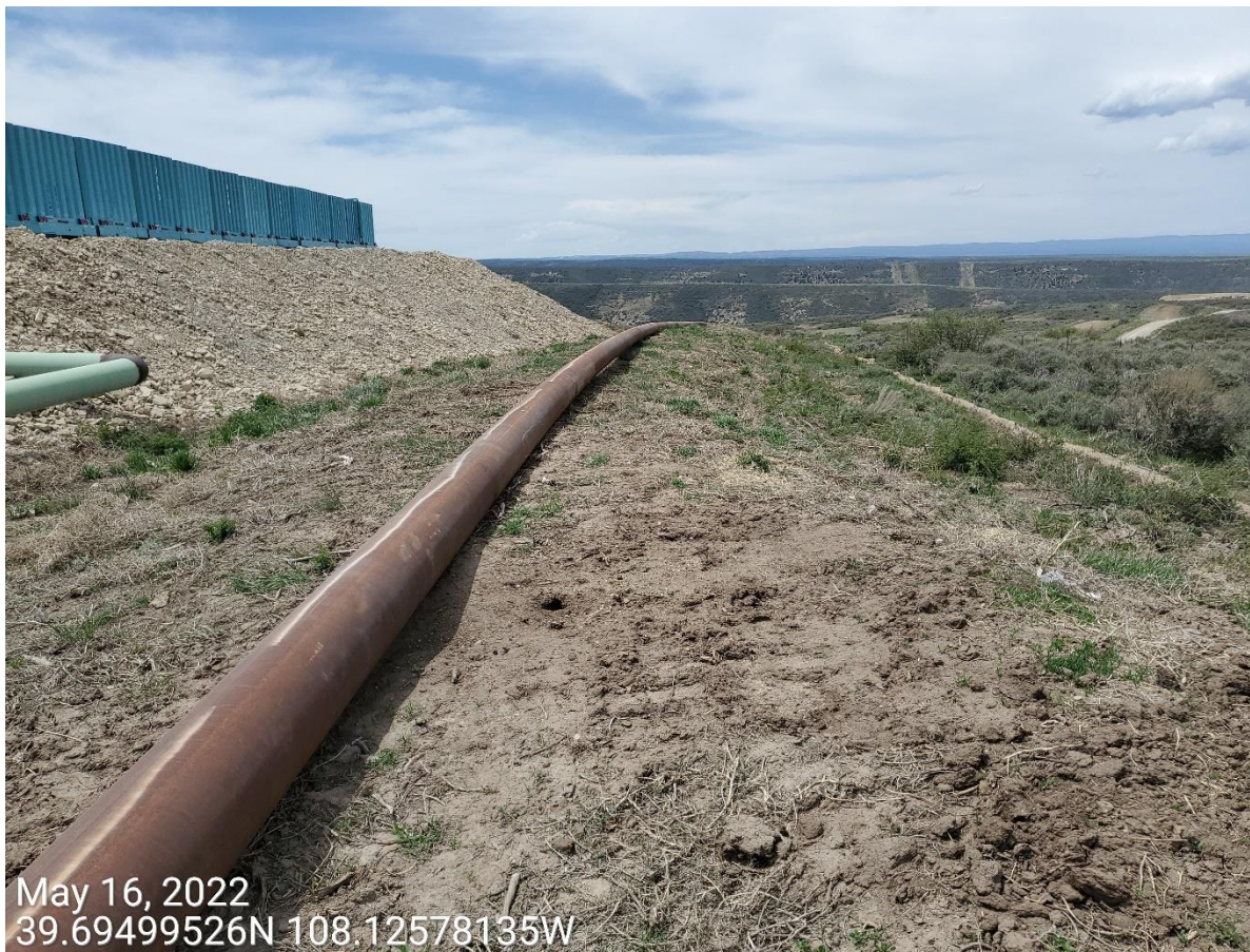
Photo 9: Photo taken from the topsoil stockpile on the north end of the Location. Photo shows Operator has constructed a pipeline that runs on the east, and north end of the Location; pipeline has been constructed directly upon the topsoil stockpiles along the perimeter of the Location. This does not appear to be protective of soils per with Rule 1002.c. Additionally, soils are exposed and at risk to erosion.
