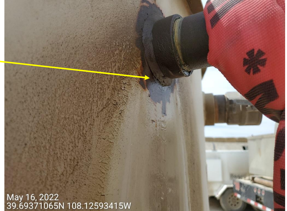
Photo 2: Fluids observed spilling from connection point of the line and tank (yellow arrow) onto the working pad surface. Stained soils also evident beneath the tank. (red arrow).
