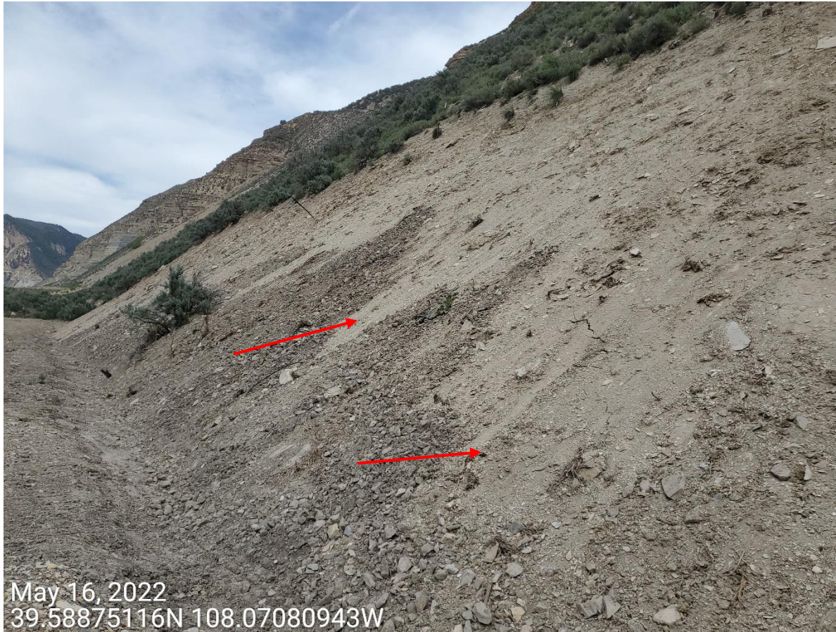
Photo 4: Photo taken from the disturbed slopes on the north end of the Location. Photo shows BMPs to minimize erosion , degradation and to stabilize the slopes have not been installed or maintained. Arrow shows example areas where additional erosion is apparent.
