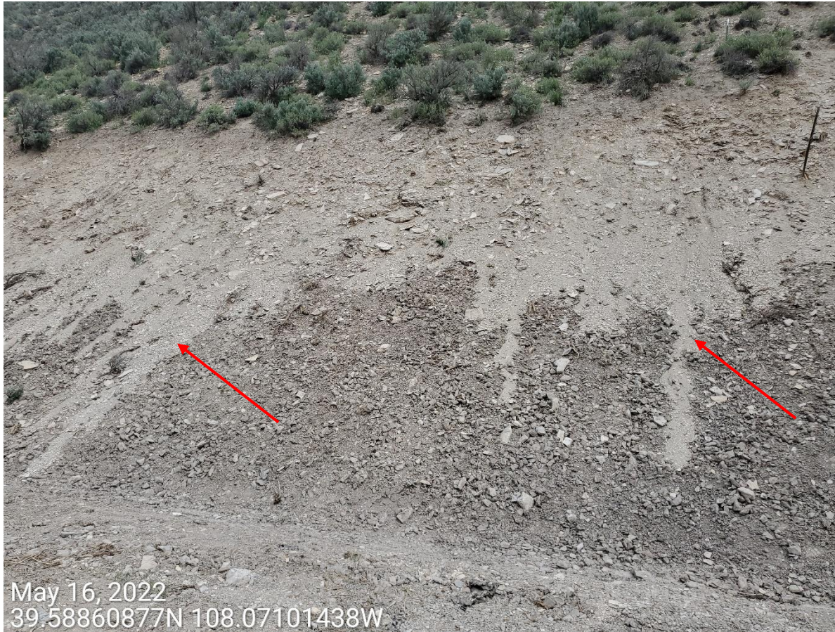
Photo 3: Photo taken from the disturbed slopes on the north end of the Location. Photo shows BMPs to minimize erosion , degradation and to stabilize the slopes have not been installed or maintained. Arrow shows example areas where additional erosion is apparent.
