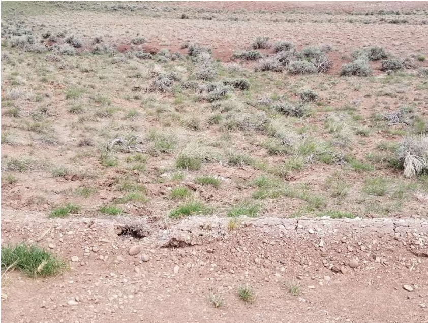
Photo 1. Breach in berm on access road where sediment is migrating off of the road.
