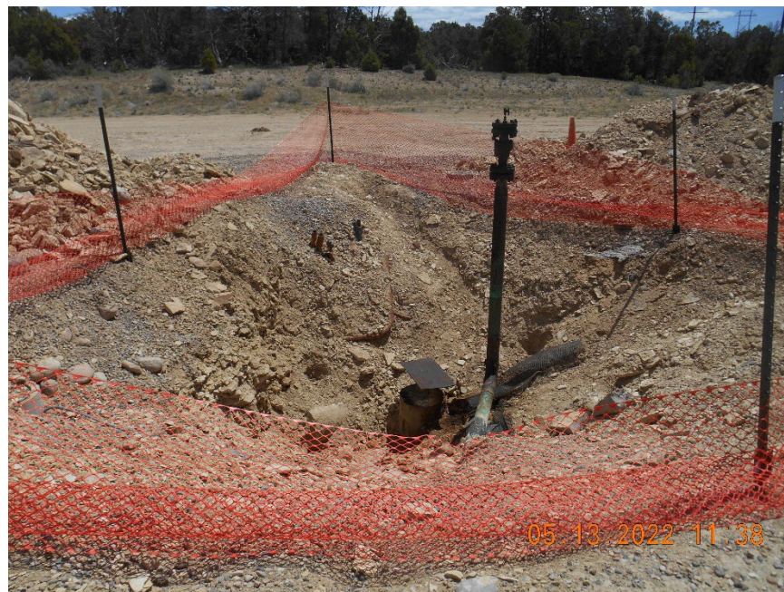
Injection wellhead Plugged and abandoned
