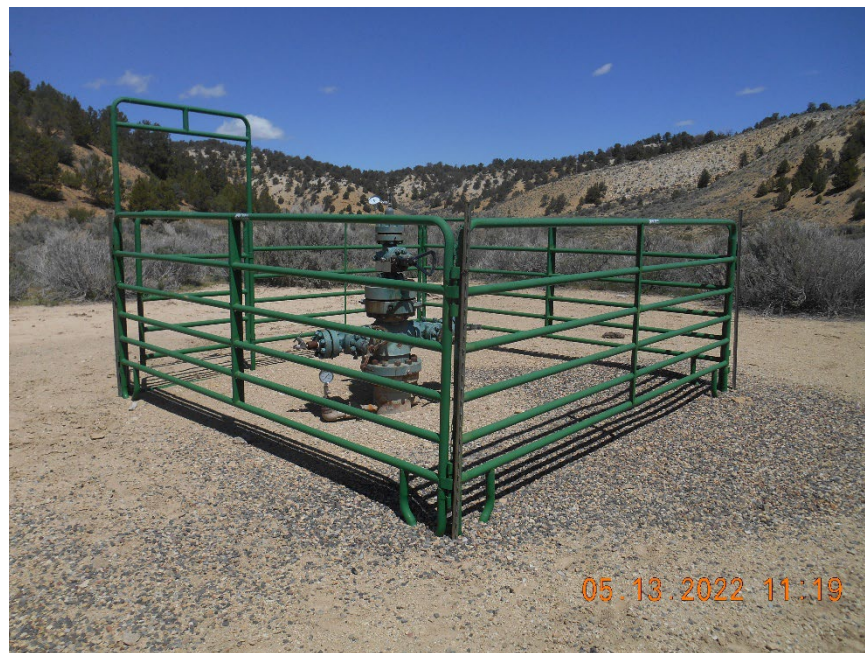
Injection Wellhead Temporarily Abandoned
