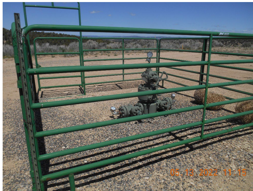
Injection Wellhead Temporarily Abandoned
