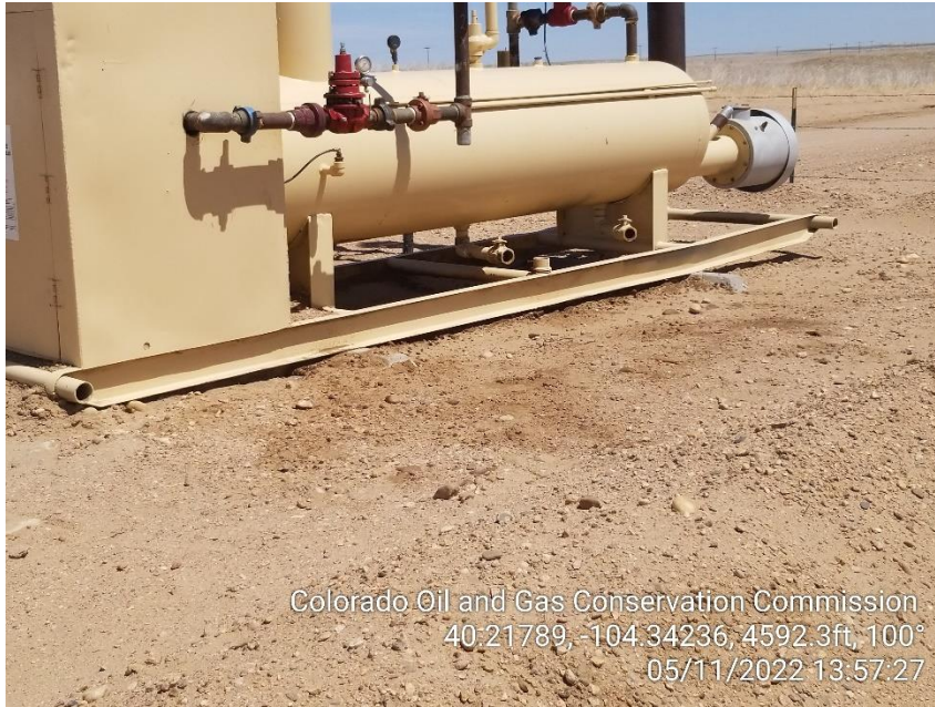
Photo 5 – Stained Soil at Separator
