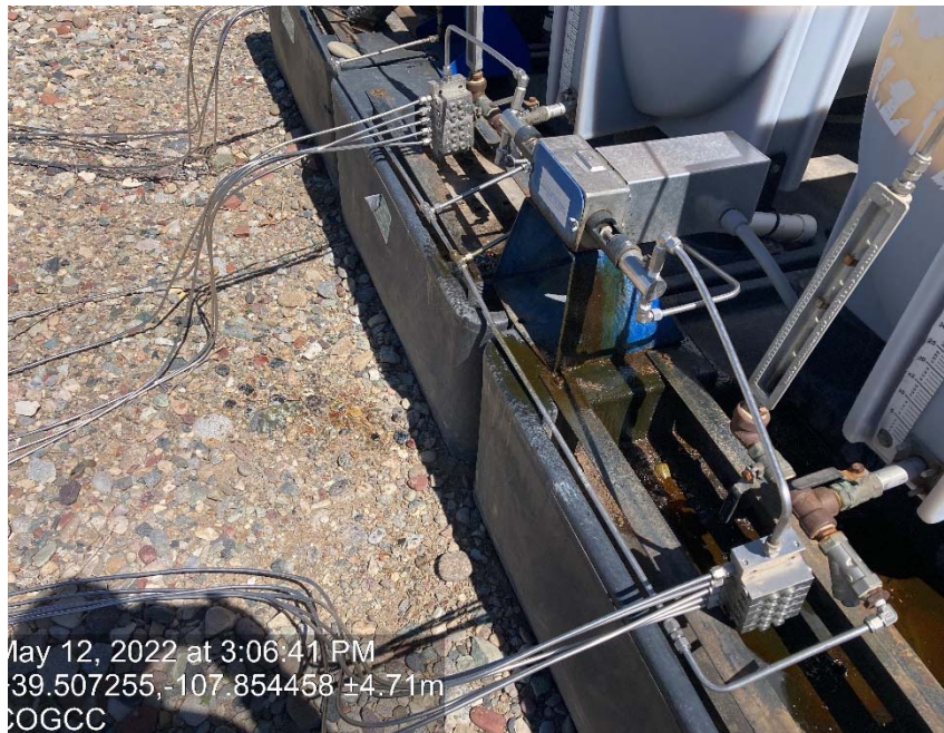
Pump leaking
