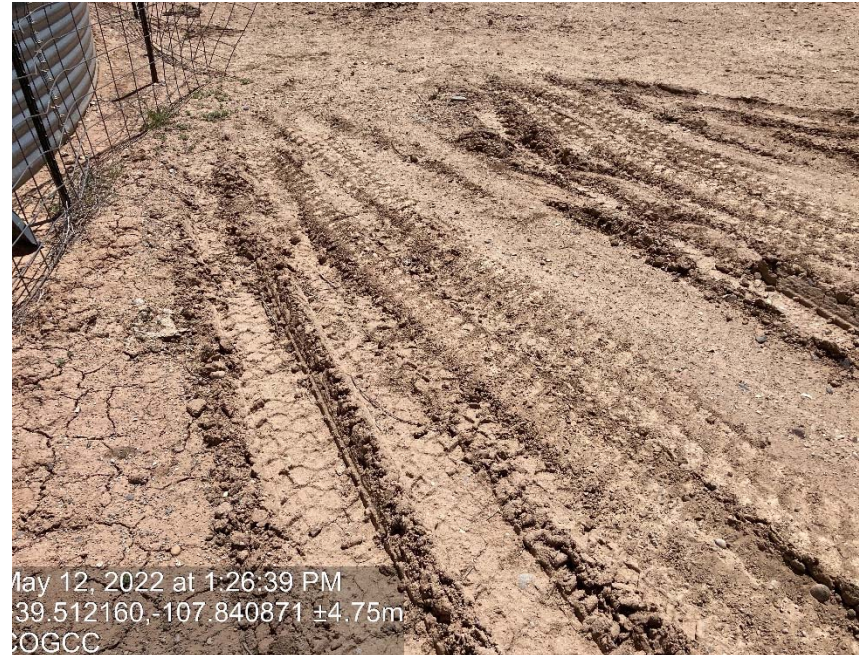
Lack of stabilization/compaction
