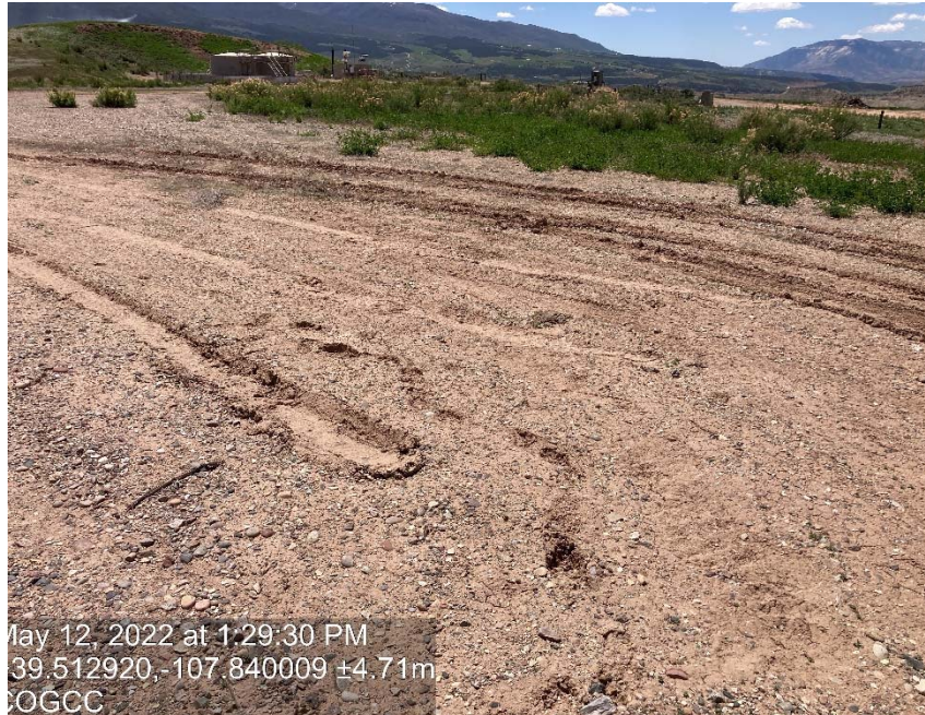
Lack of stabilization/compaction
