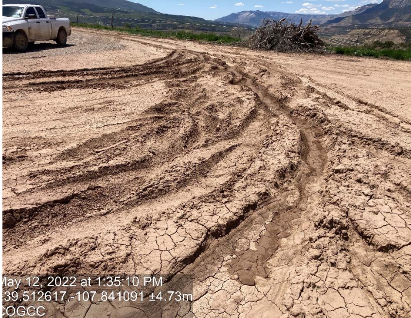
Lack of stabilization/compaction
