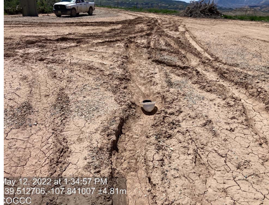
Lack of stabilization/compaction
