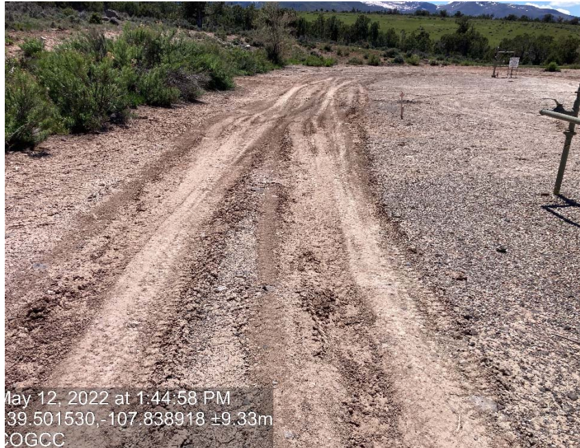
Lack of stabilization/compaction
