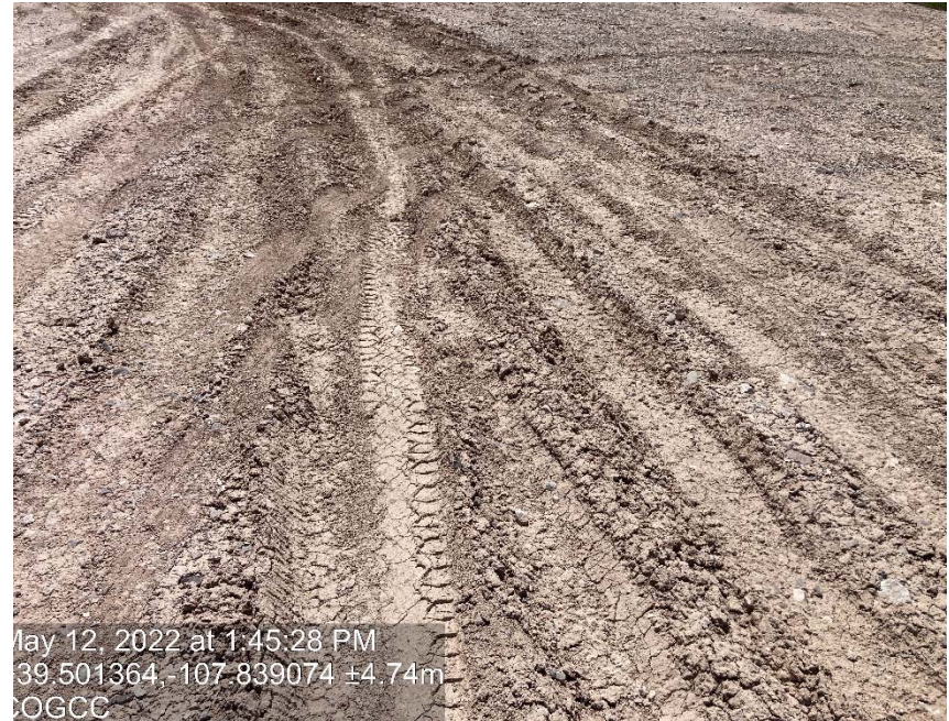
Lack of stabilization/compaction
