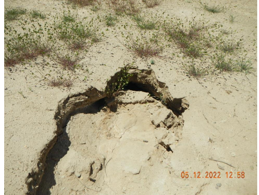
Subsidence of ground behind tank battery.
