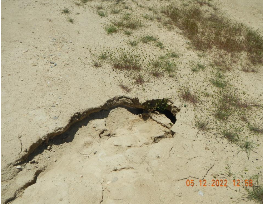
Subsidence of ground behind tank battery.
