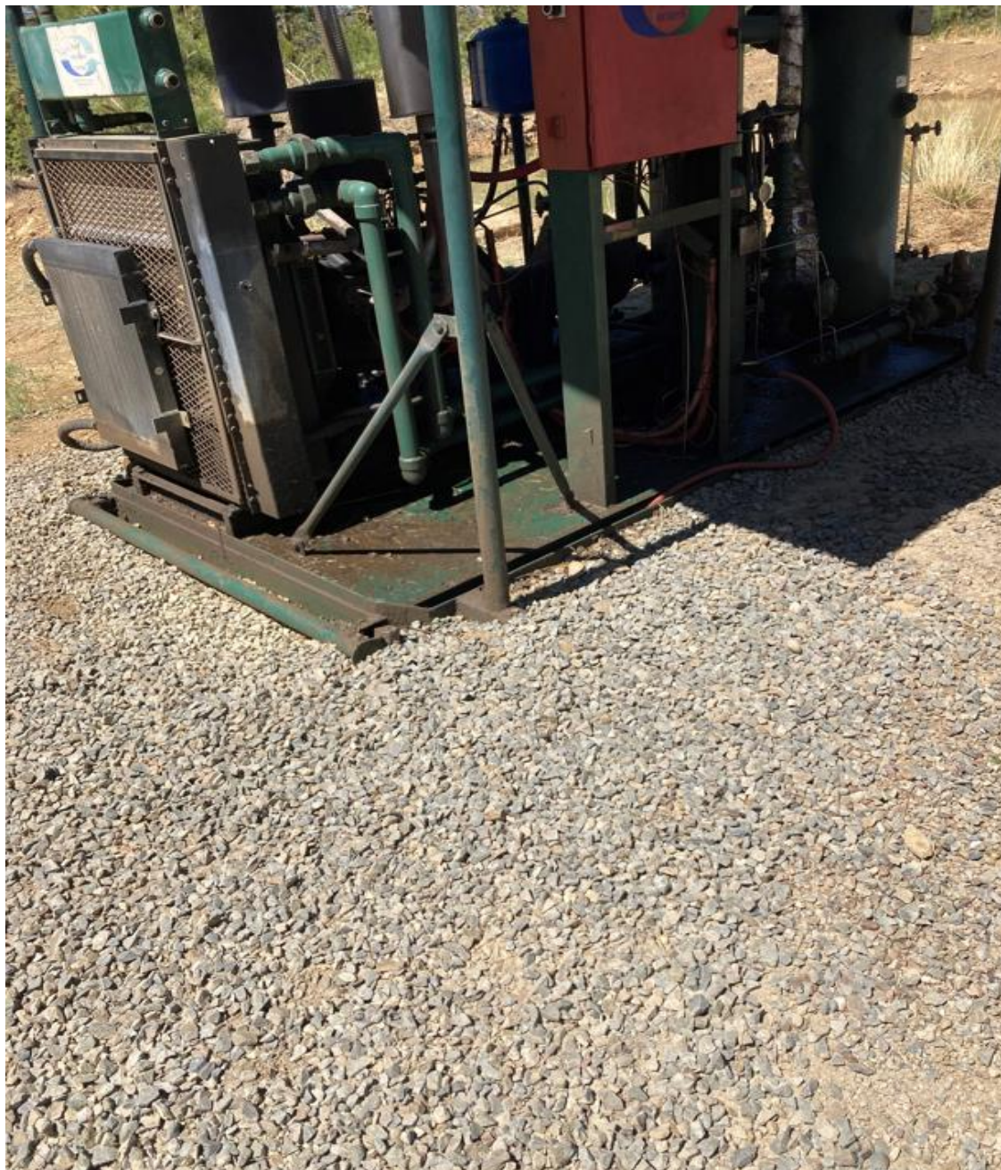
PHOTO 1: MAINTENANCE HAS BEEN PERFORMED AND THE ENGINE SKID HAS BEEN CLEANED. THE IMPACTED SOIL AROUND THE SKID WAS CLEANED UP AND REMOVED FROM LOCATION AND THE SELF INSPECTION PROCESS HAS BEEN REVIEWED. THE LEAK ON THE PRODUCED WATER TANK HAS BEEN FIXED, ALL VALVES, PIPES, AND FITTINGS HAVE BEEN SECURELY FASTENED TO ENSURE GOOD MECHANICAL CONDITION.
