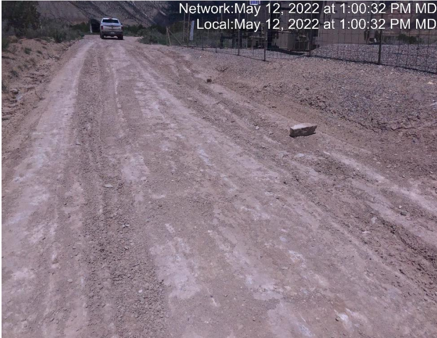
Photo #6692 Insufficient tracking BMP at entrance to location.
