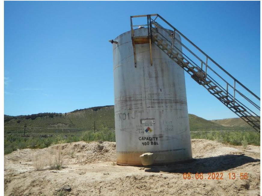
**Berm has weeds growing inside of it. Walls and base need maintained.**
