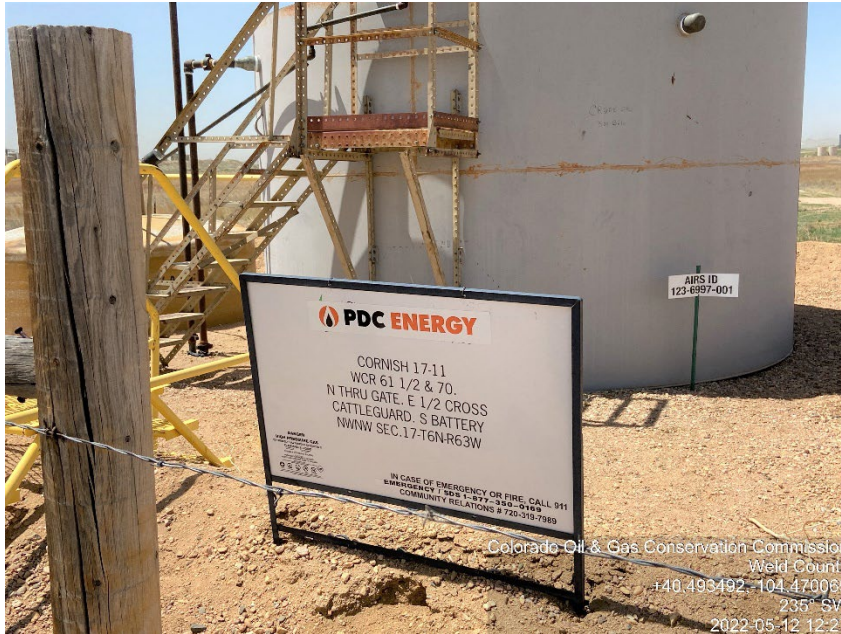
Photo #5 Cornish 17-11 Battery site Active Battery sign
