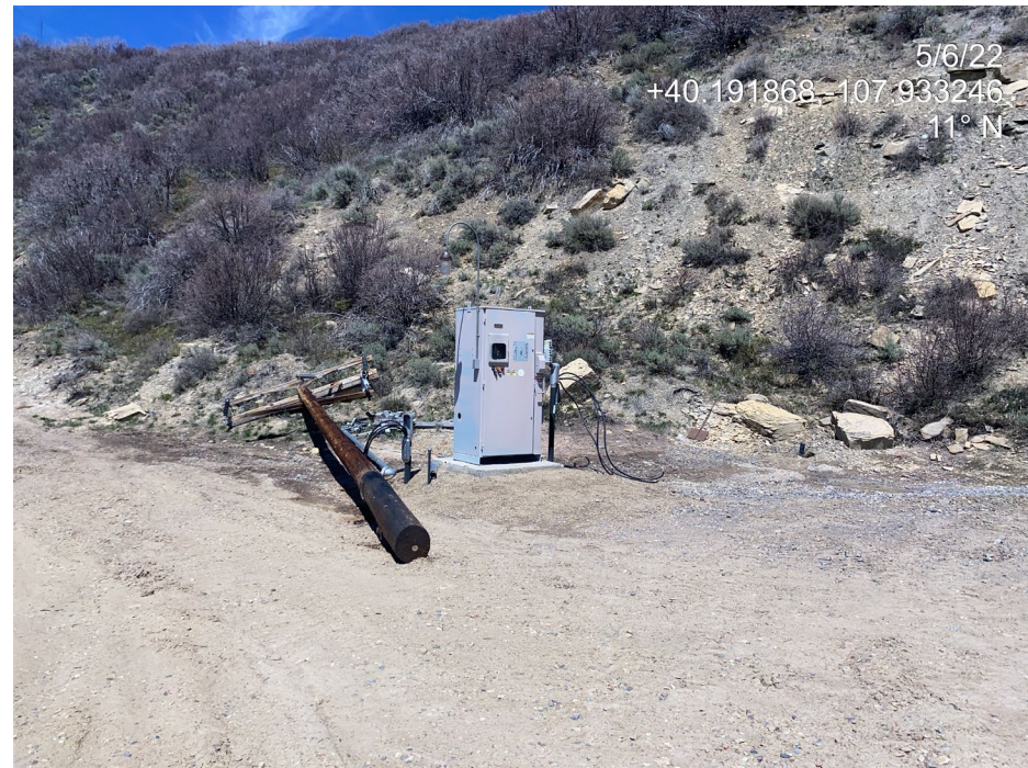
Photo 6. Photos shows power lines being decommissioned at the Location.
