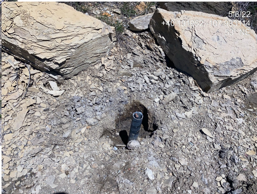
Photo 4. Photo taken from the north of the Location shows buried electrical lines which will need to be removed.
