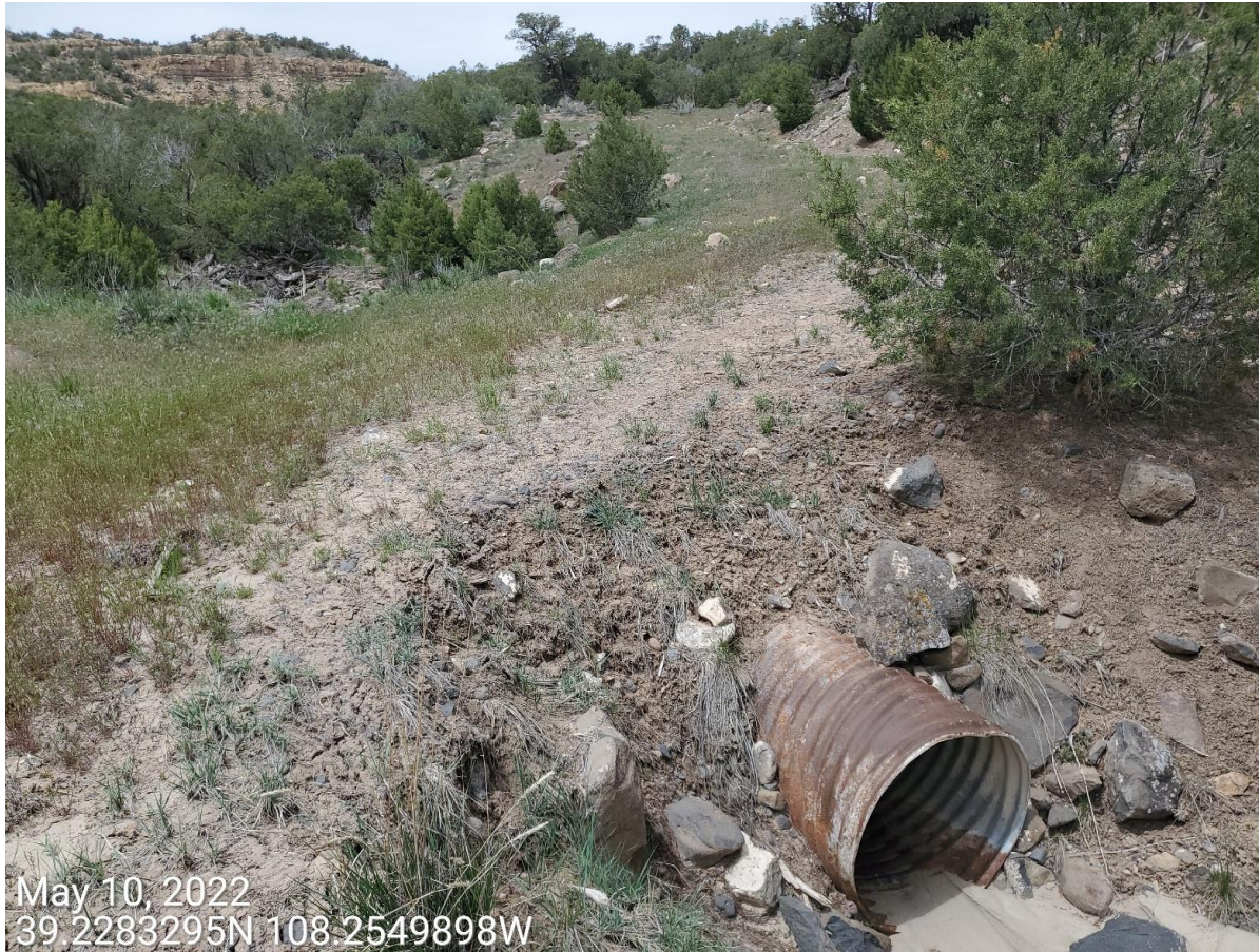
Photo 7: Photo example showing culvert remaining at access road.
