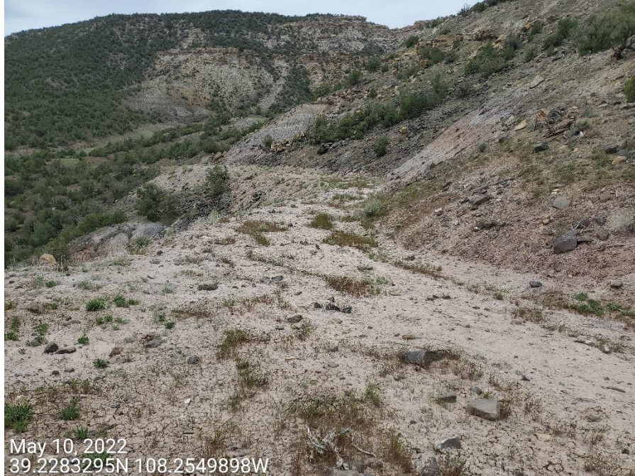
Photo 6: Photos examples showing remaining access road has not been recontoured/regraded and reclaimed in accordance with 1004 rules.
