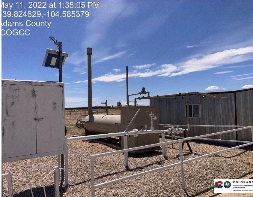
Pic 2 gas meter run, separator, locked shed
