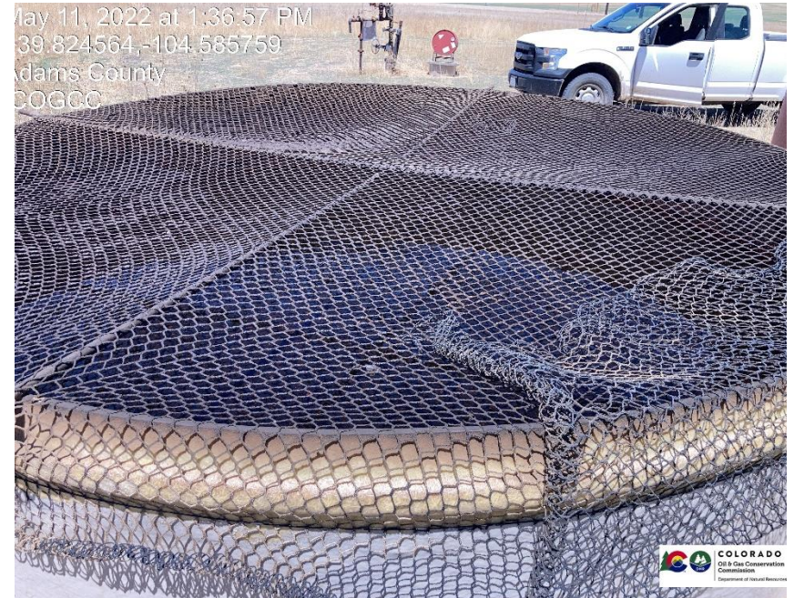
Pic 4 open top tank is approx. 2' from overflowing, precipitation may cause a spill.
