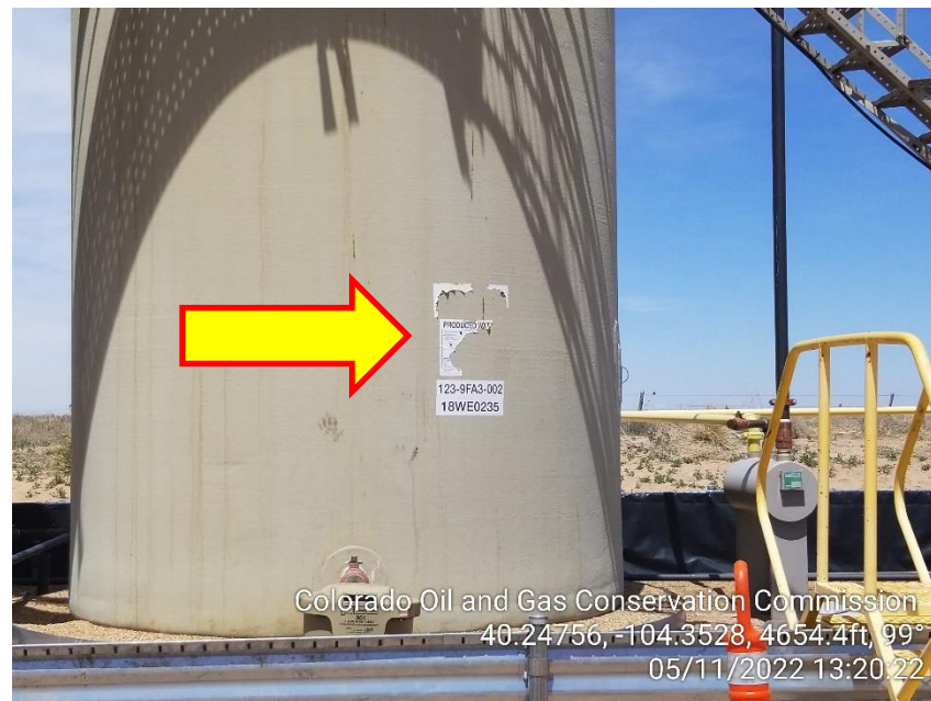
Photo 4 – Labels missing on Produced Water Tank
