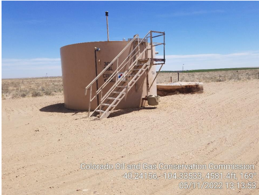
Photo 5 – New Tank installed – No Berms
