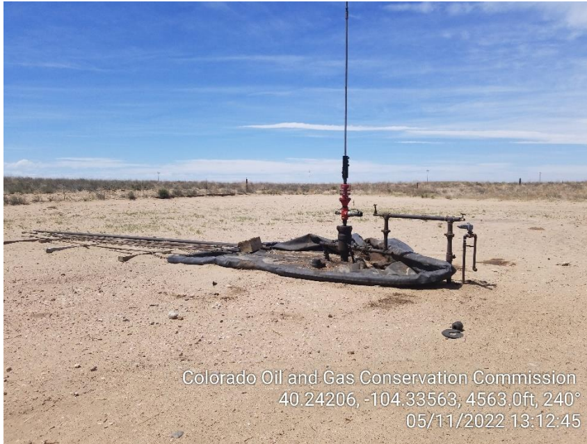
Photo 1 – Wellhead – Unused Rods and Stained Soil
