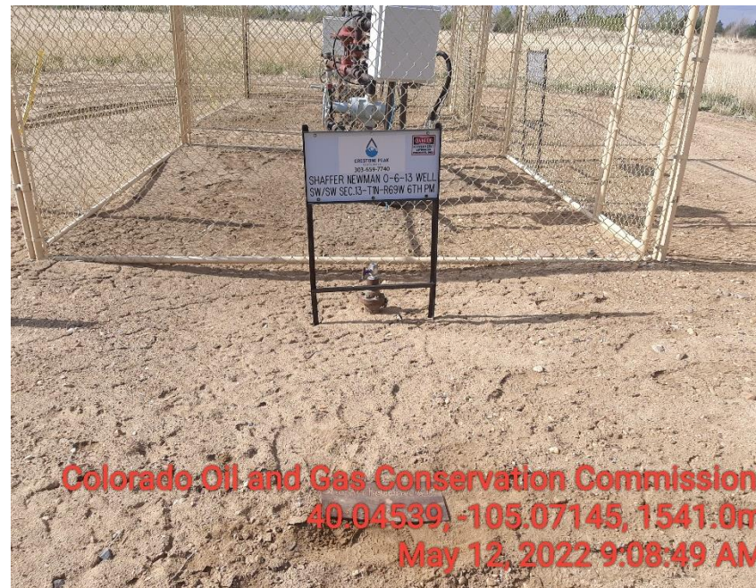
Photo 2 P&A well unmarked not LOTO riser.
