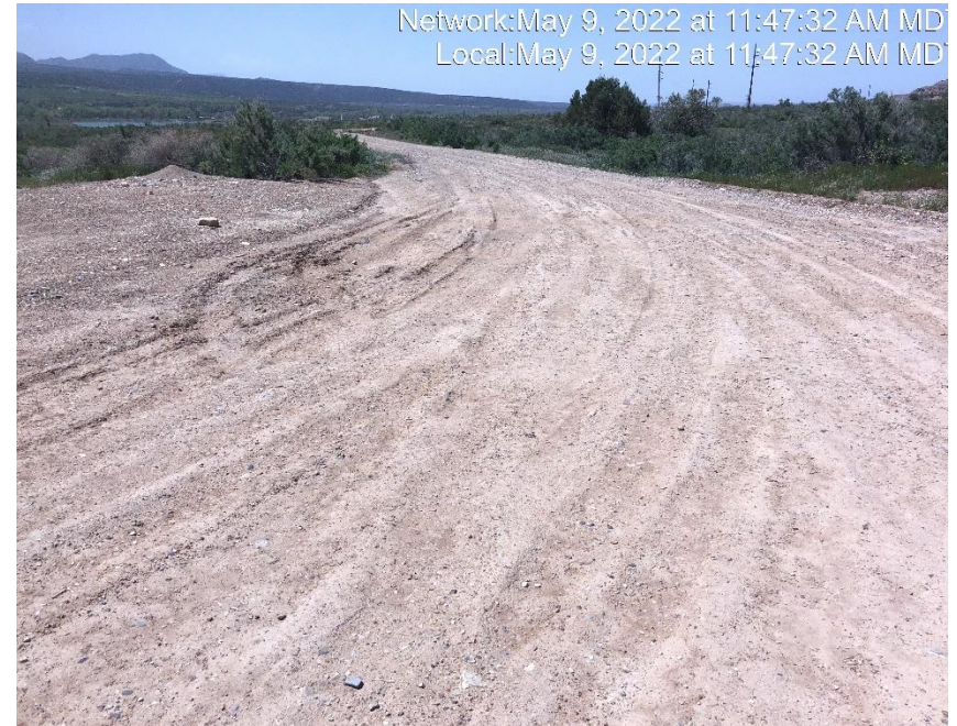
Photo #6644 Insufficient tracking BMP at entrance to location.
