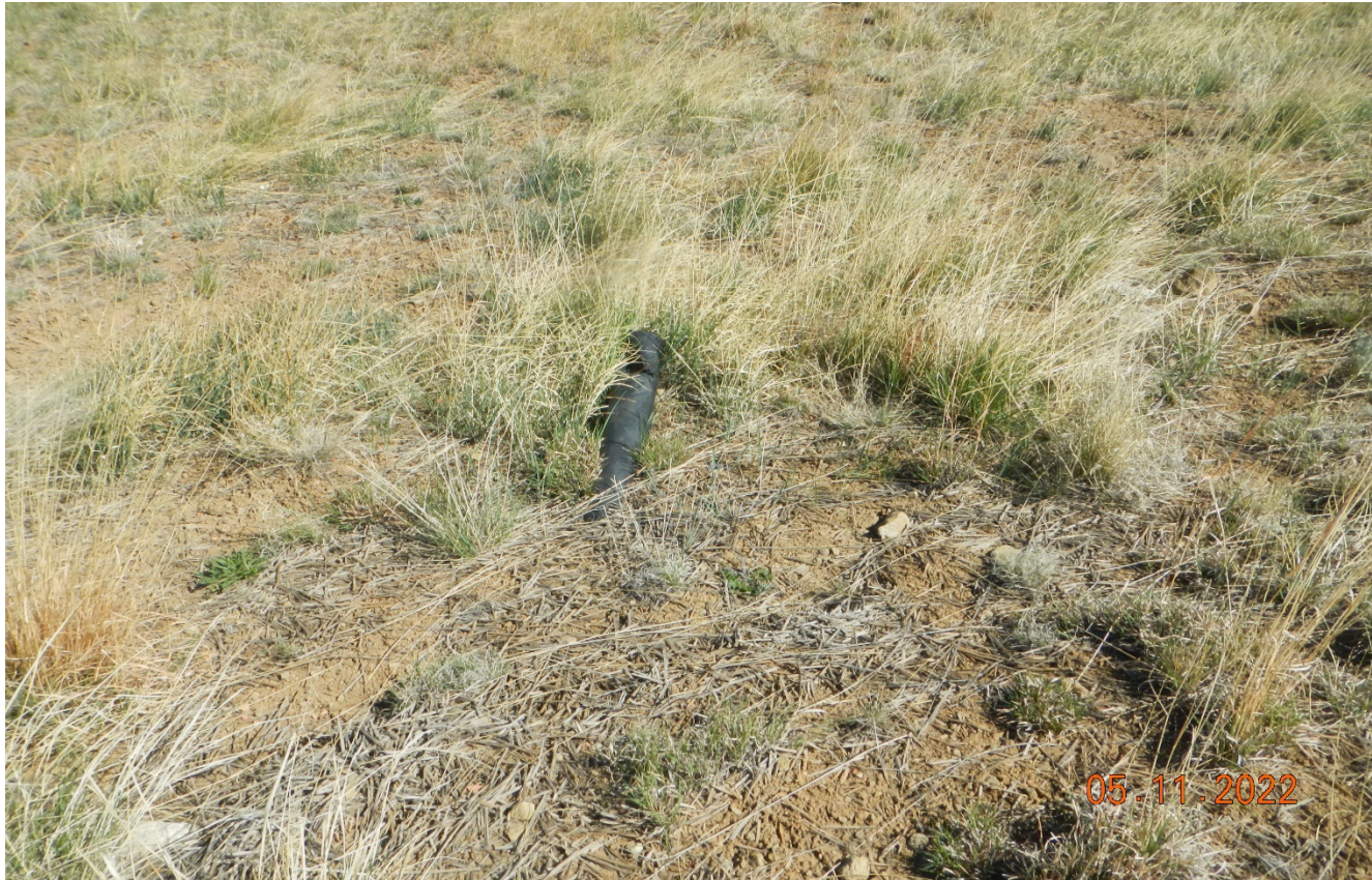
Photo 3. There is a black pipe sticking out of the fill slope at the location.
