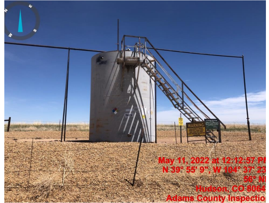
Photo#2 Production Tank
