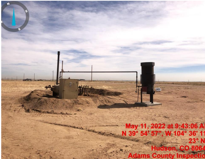
Photo#5 Separator and ECD
