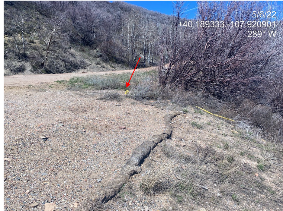
Photo 6. Photo taken at the east of the Location shows a straw wattle is no longer in proper functioning condition. Sediment was observed to have moved over the wattle. Note also the unmarked anchor (red arrow).
