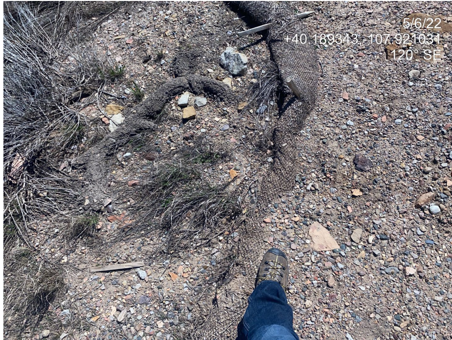
Photo 5. Photo taken at the east of the Location shows a straw wattle is no longer in proper functioning condition. Sediment was observed to have moved over the wattle.
