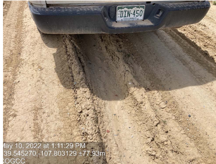
Lack of stabilization/compaction/ degradation
