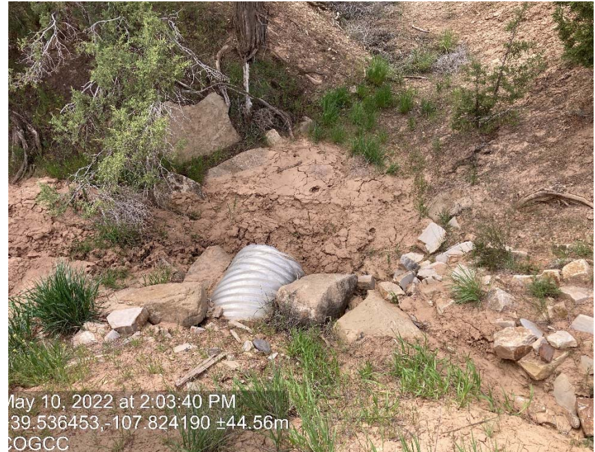
Erosion at culvert
