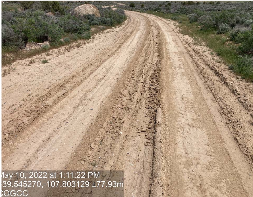
Lack of stabilization/compaction/ degradation
