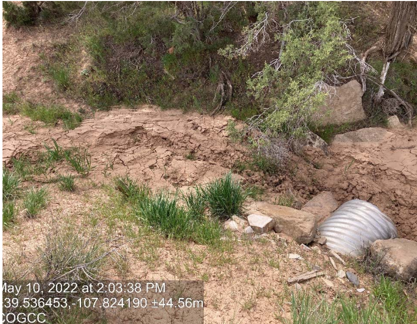
Erosion at culvert
