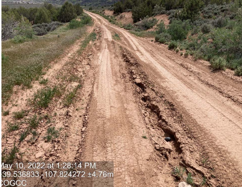
Lack of stabilization/compaction/ degradation
