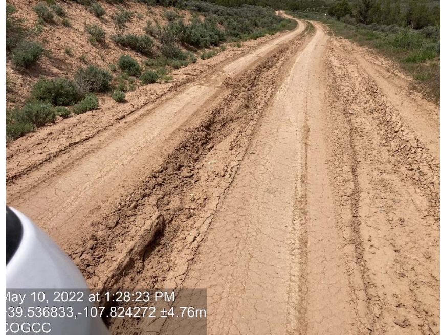
Lack of stabilization/compaction/ degradation
