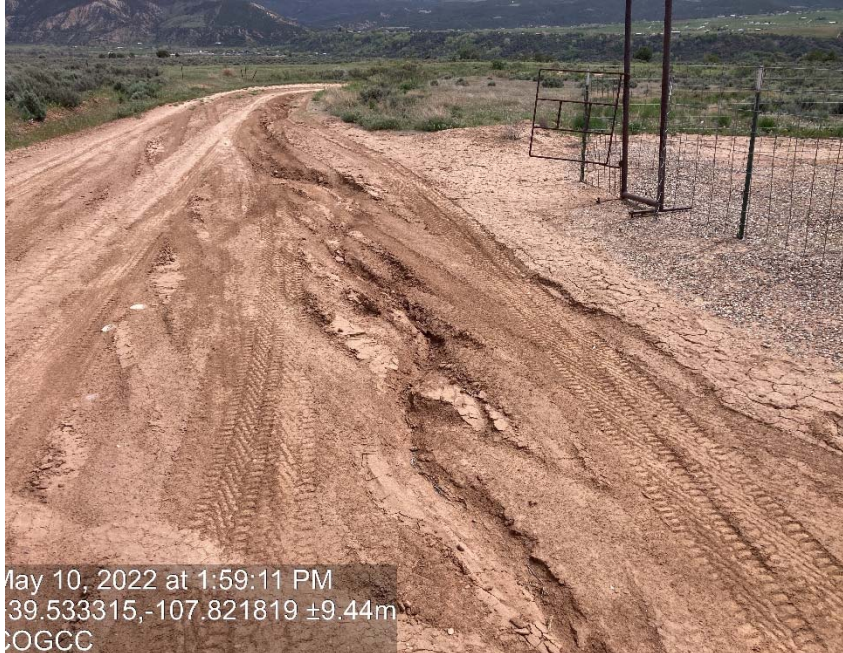
Lack of stabilization/compaction/ degradation
