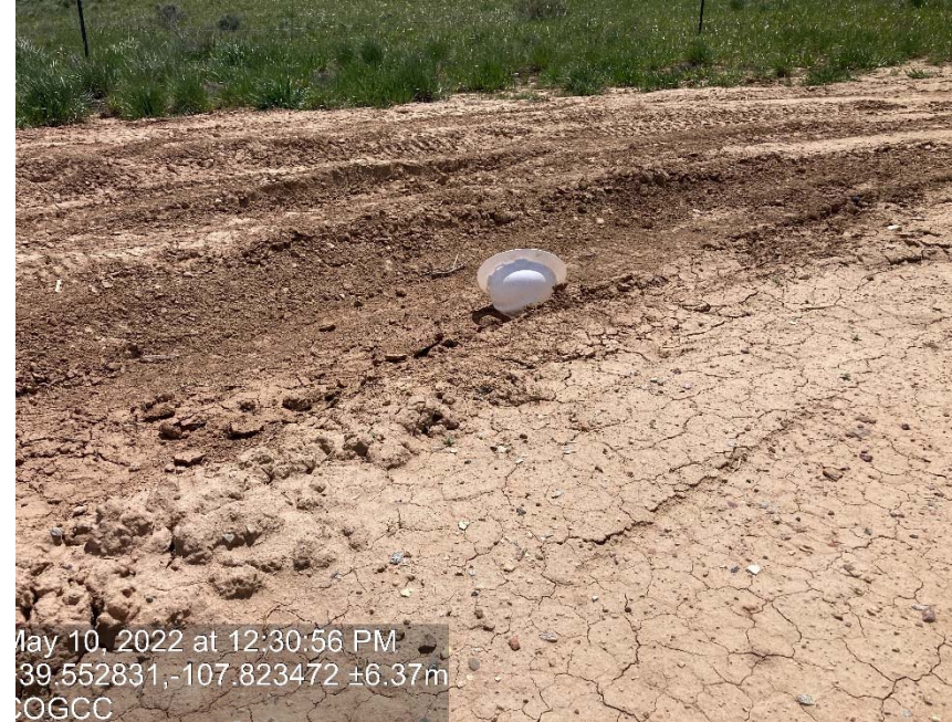
Lack of stabilization/compaction
