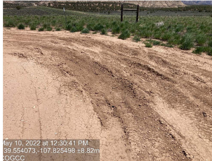
Lack of stabilization/compaction
