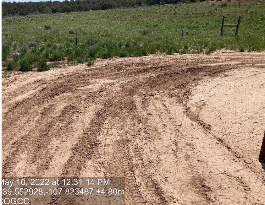
Lack of stabilization/compaction
