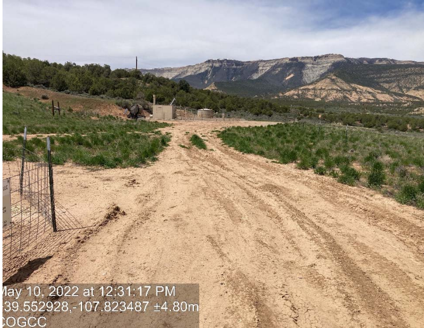
Lack of stabilization/compaction
