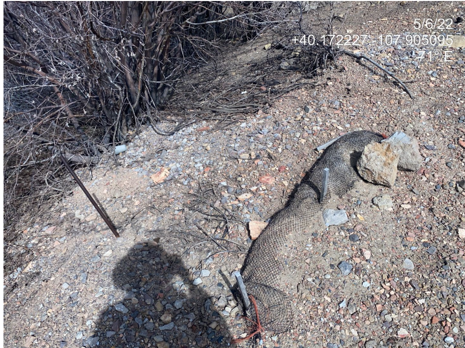
Photo 5. Photo shows a properly functioning straw wattle. In other locations at the northwestern edge of the Location erosion was occurring resulting in soil movement offsite.
