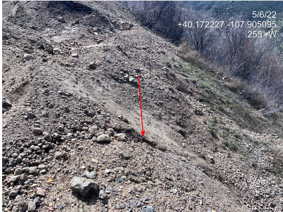
Photo 3. Photo shows piles of excavated material at the edge of the Location. No BMPs were observed to prevent soils potentially contaminated with E&P waste from migrating off the Location. Also note the rill occurring (red arrow) due to inadequate stormwater controls.
