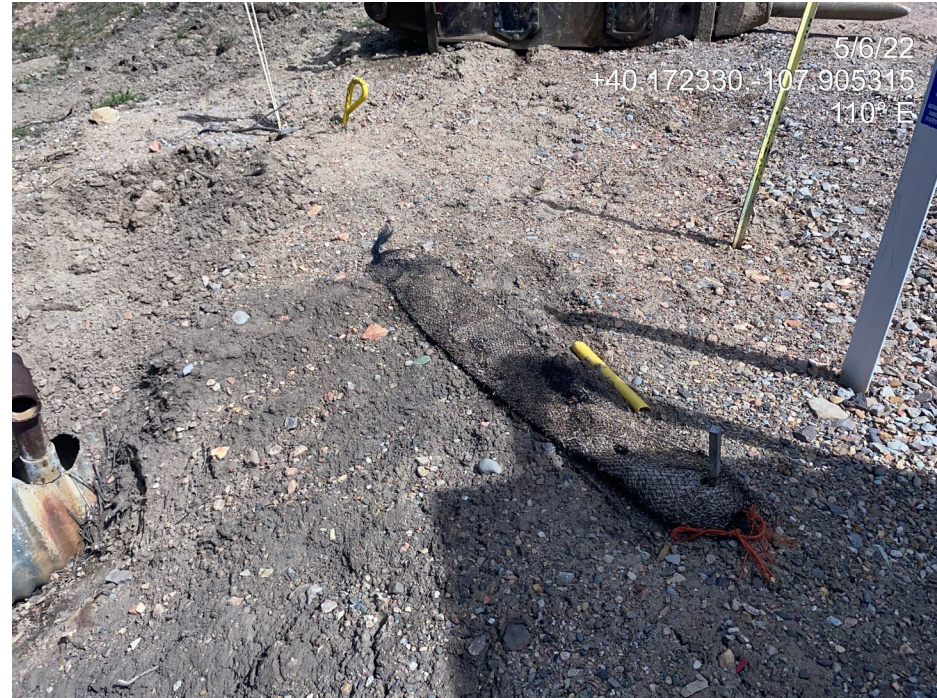
Photo 6. Photo shows a straw wattle not properly maintained. Some erosion was occurring at the edge of the Location resulting in soil movement offsite.
