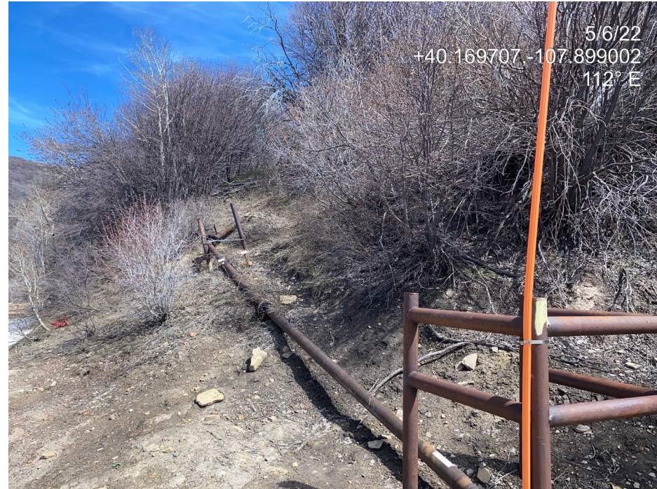
Photo 2. Photo shows flowlines adjacent to the Location which will need to be removed for final reclamation. Note, GPS coordinates are incorrect due to phone GPS malfunction.
