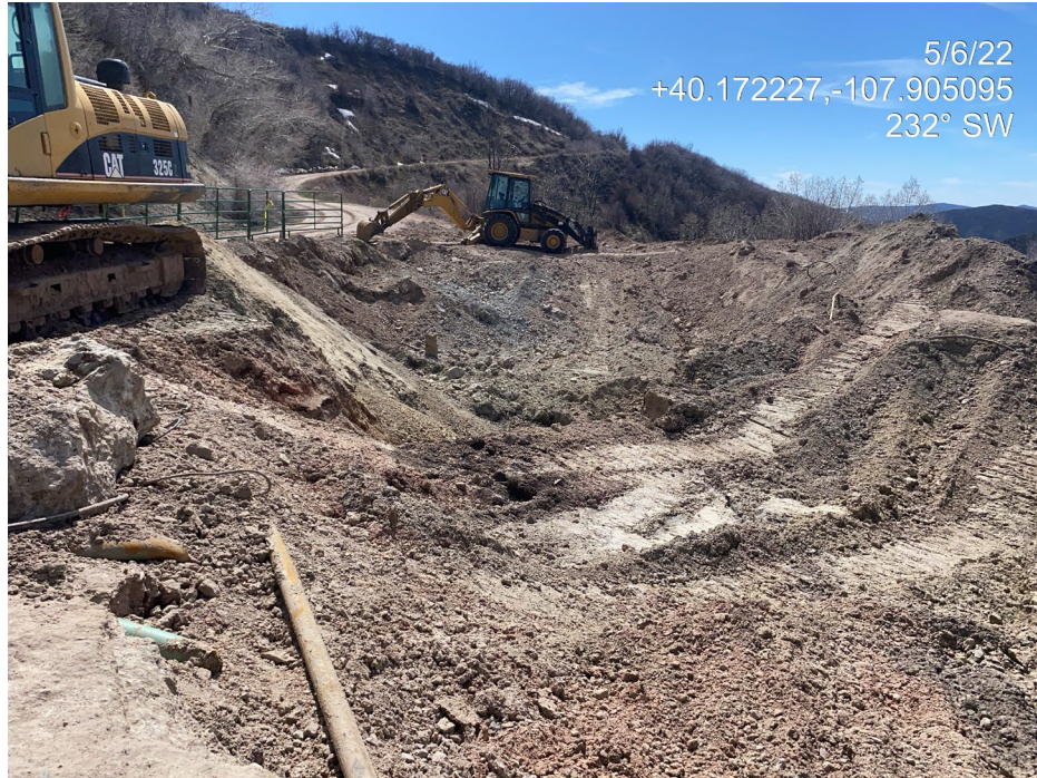
Photo 1. Photo taken from the well area shows the excavated area around the well. Photo also shows multiple underground pipes and flowlines which will need to be removed for final reclamation.
