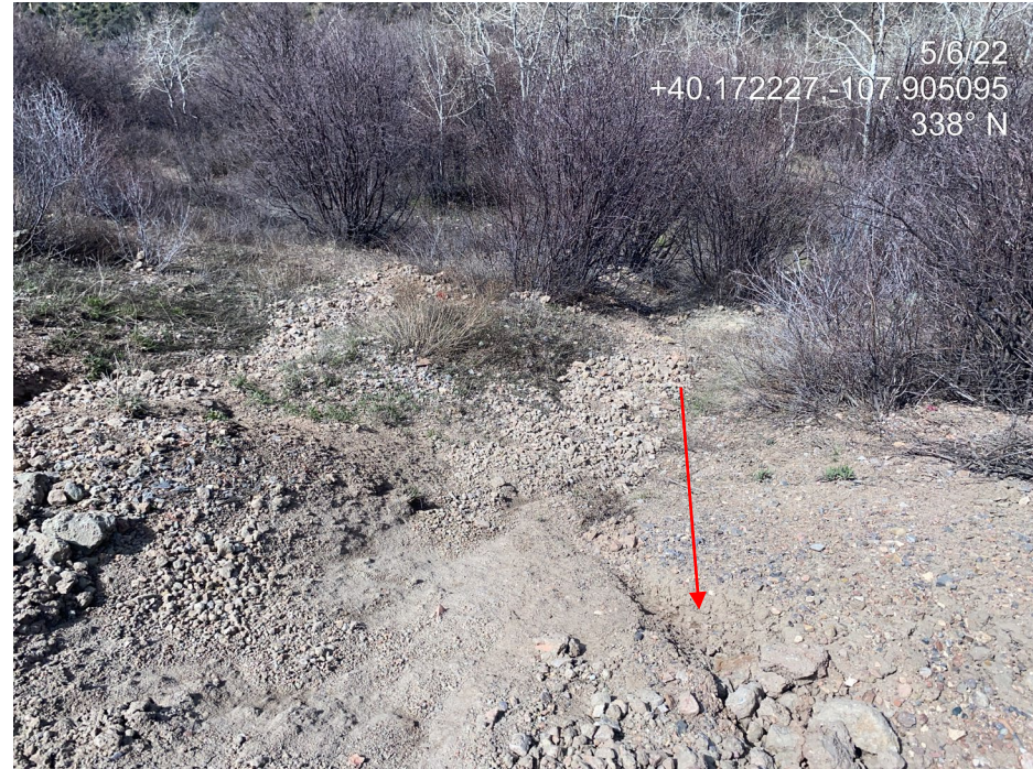
Photo 4. Photo shows a rill occurring (red arrow) due to inadequate stormwater controls. Photo also shows sediment and gravel from the Location is present offsite.
